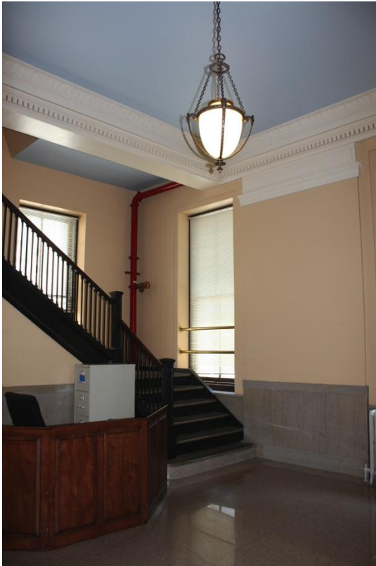
Figure 17: eleventh fixture, NW corner postal lobby
