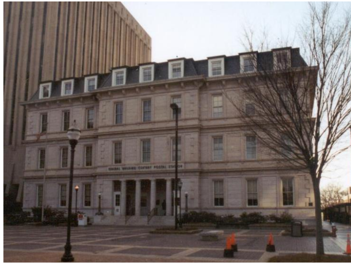
Figure 6: View of front or east elevation, 2005
