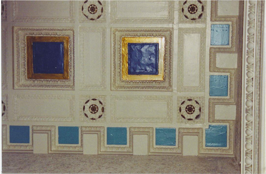
Figure 13: Corner detail of courtroom ceiling, 2005
