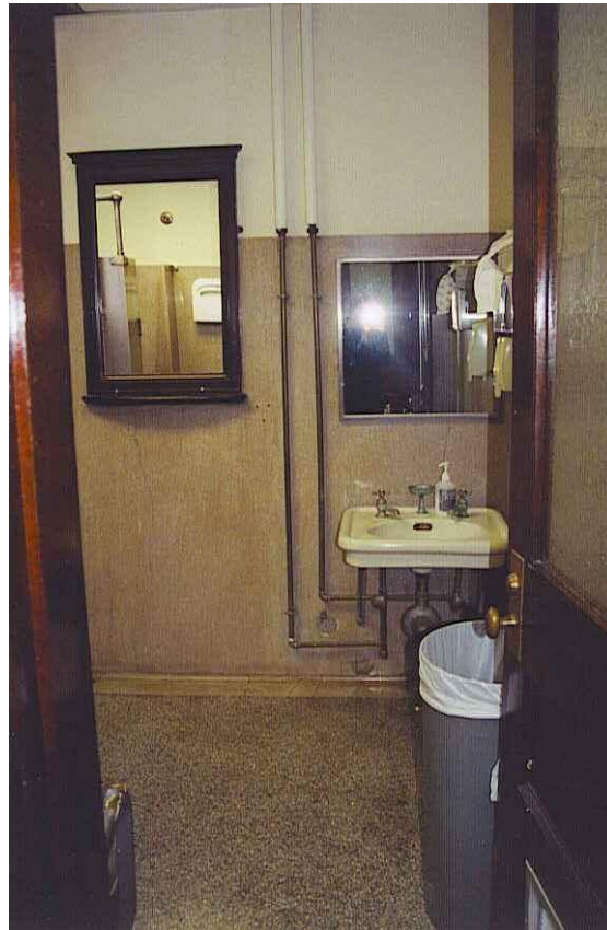
Figure 14: Example of second and third floor bathroom
