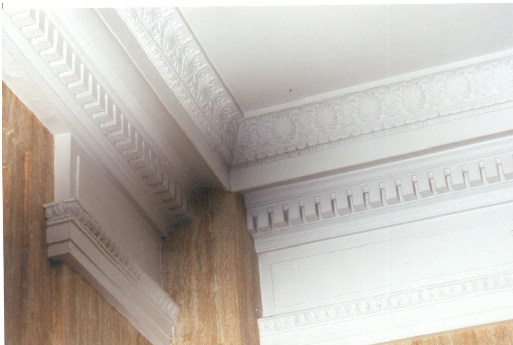
Figure 9: Detail of lobby plaster work, 2005
