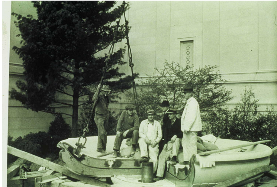
Figure 20. Tennessee pink marble fountain being assembled on site, National Gallery of Art, circa 1940. Courtesy Knox County Public Library, McClung Historical Collection, Barksdale Jones images.
