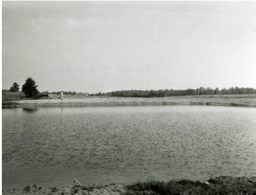
Figure 7. Man-made pond , 10-01-59. Photographer's notes: "Pond constructed in the spring of 1959 under Soil Bank program. Pit-type pond 150 feet square and 6 feet deep, with 4:1 side slopes. Pond is constructed on Dickson soil. Located eight miles south of Woodbury." Photographed by: W.L. Clement. Source : Cannon County, Tennessee Farms, Walker Library at MTSU, Digital Collections.
