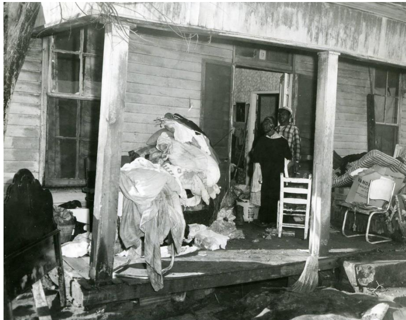
Figure 23. Home destroyed in flood , 03-13-1963. Photographer's notes: "One of several homes flooded in city limits of Woodbury from floodwater of Stones River. Water got about three feet deep in this house. Contents damaged and some destroyed." Photographed by W.L. Clement. Source : Cannon County, Tennessee Farms, Walker Library at MTSU, Digital Collections.
