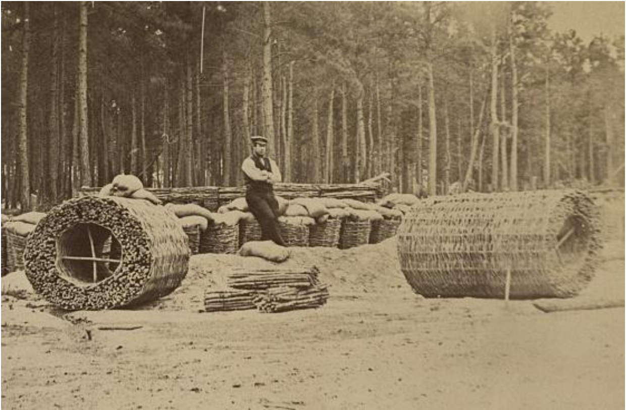
Fig. 3.1. Gabions and Fascines
