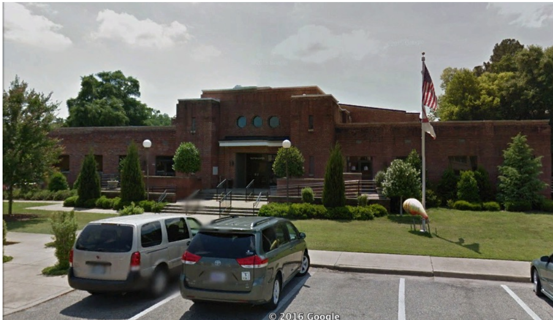
Figure 32 - 2015 view of the Doster Memorial Community Center, which was built by the WPA as a National Guard Armory. Image courtesy of Google Earth.
