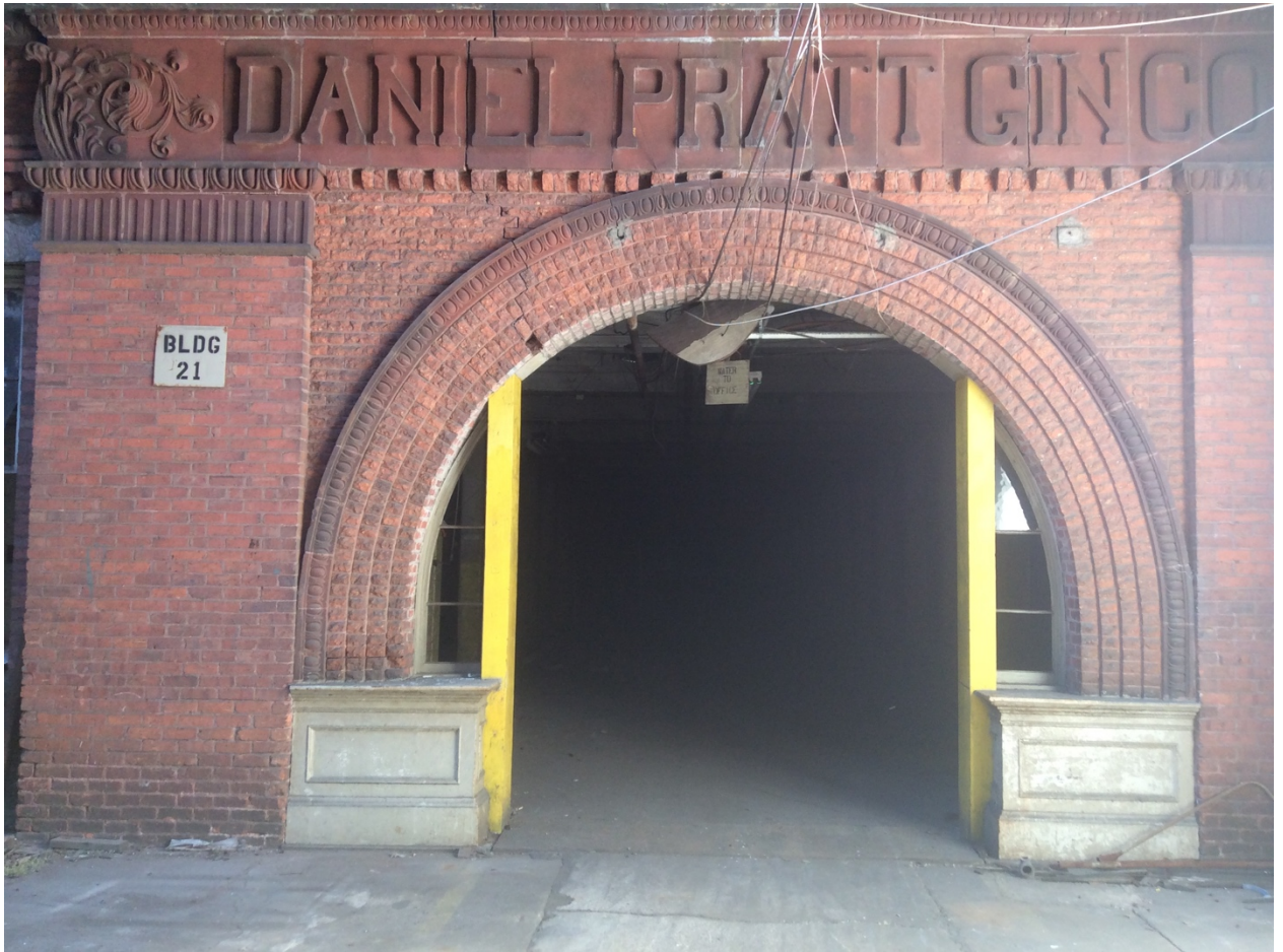
Figure 14 - Detail of Syrian arch and raised terra cotta lettering on front of 1896 building.
