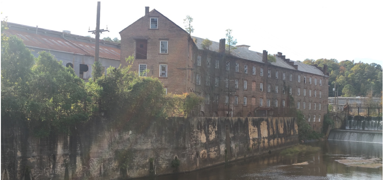
Figure 22 - View of damage to sash, door, and blind factory building. Note smashed windows, trees and other vegetation growing on building.
