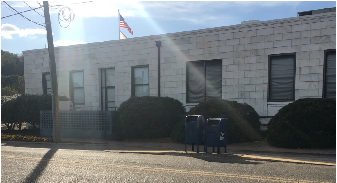
Figure 38 - USPS drop off boxes located on the eastern side of the City Hall Annex.
