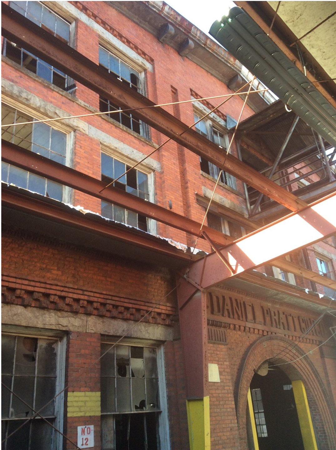
Figure 21 - View of damage to 1896 building.
