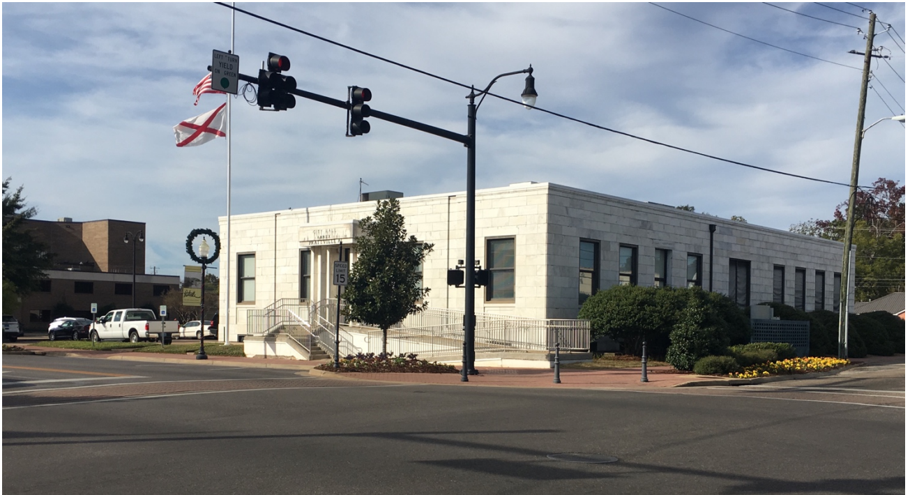
Figure 34 - View of City Hall Annex, formerly the Prattville post office, from the southeast.
