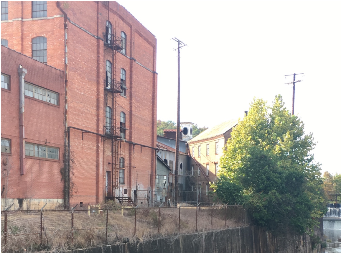
Figure 11 - View from Autauga Creek of junction of sash, door, and blind factory building with later additions to complex.
