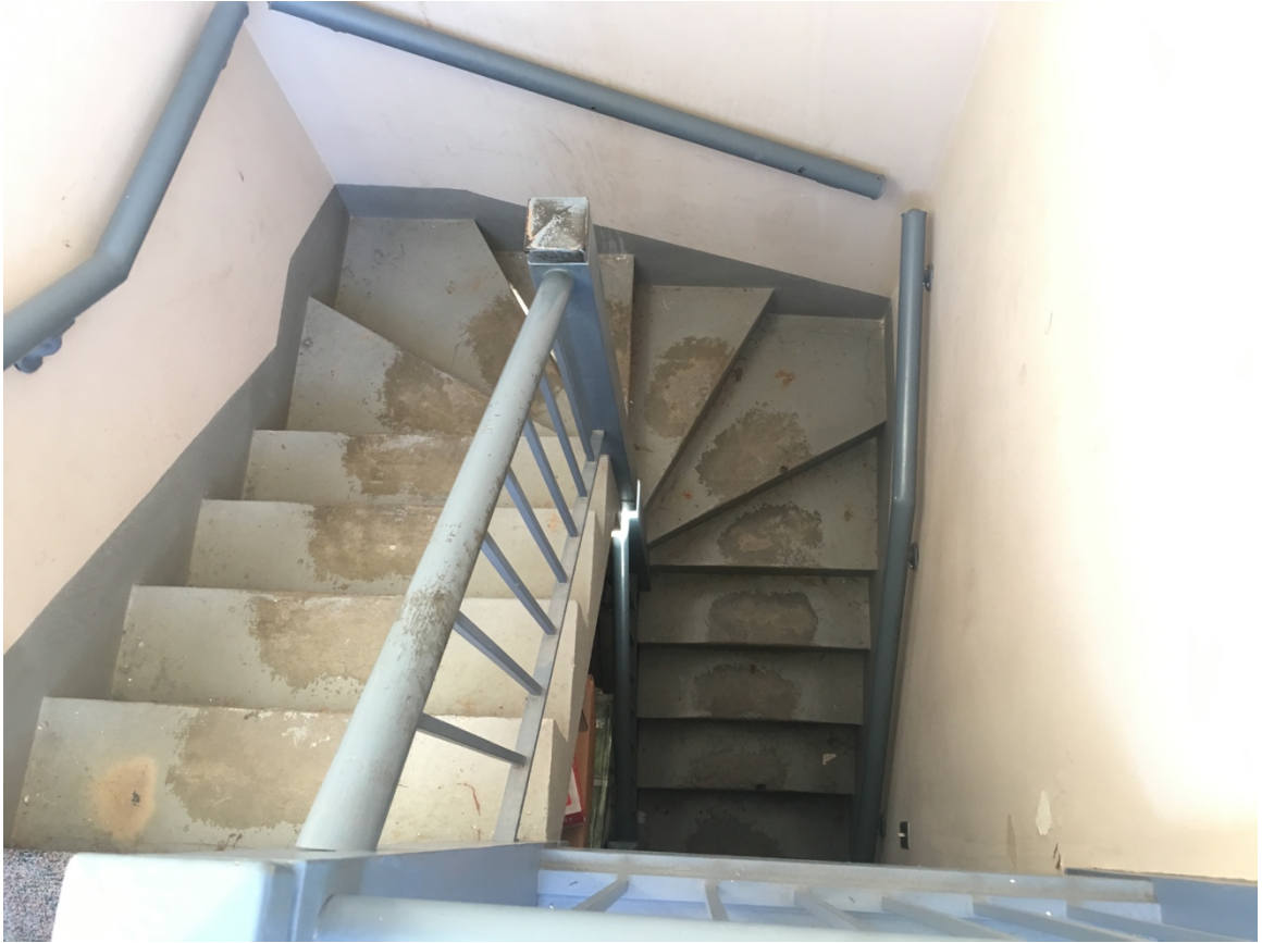
Figure 39 - Interior detail of original staircase in City Hall Annex.
