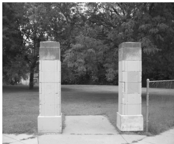
Figure 29: Rodney Crowley Playground Entrance.
