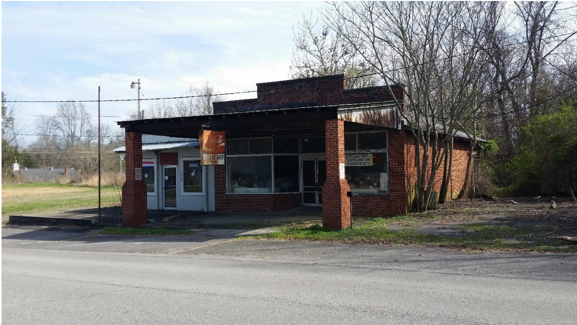
Figure A.18 Abandoned gas station and post office. The buildings are located at the crossroads of McMinnville Highway and Quebeck Road. Photo taken by author.
