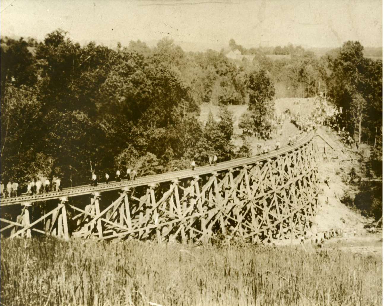
Figure 2.13 N&ATLC Railroad trestle crossing through Crain Hollow. The trestle is under construction. Photograph courtesy of Heritage Alliance of McMinnville.
