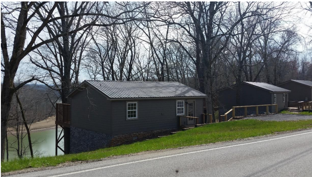
Figure A.17 New cabins have been built recently in Walling along the original route of the Memphis-to-Bristol Highway. The cabins overlook the Caney Fork, which can be seen in the background. Photo taken by author.
