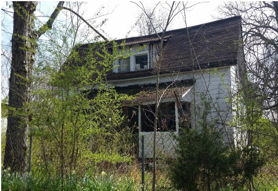
Figure A.13 RRC&L Company house on Solomon Street, abandoned. Photo taken by author.
