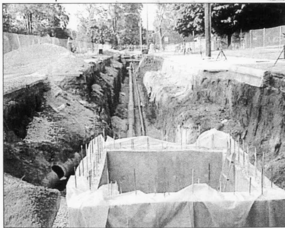
Photo by James Evans | Managing Editor This trench behind Rutledge Hall was dug to accommodate the replacement of old steam lines with new ones. Officials in the Construction Administration Office are hoping this leg of the project will be completed before the fall semester.
