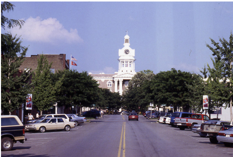
Figure 7. “The Public Improvement Project buried electric lines, renovated sidewalks and streets, and added period lighting and landscaping.” 58
