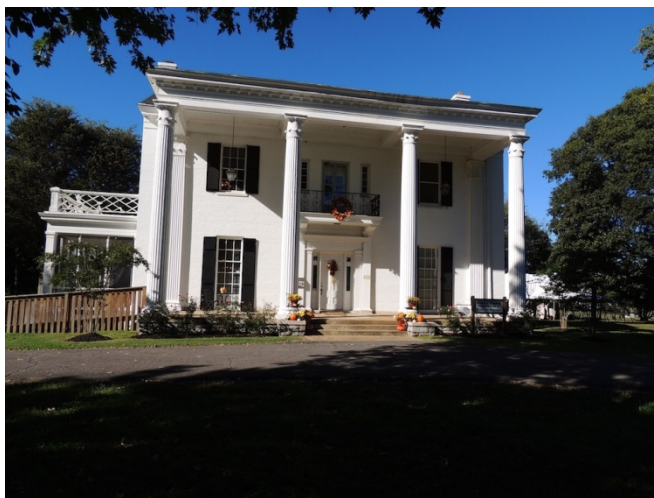
Figure 13. The Comer House
