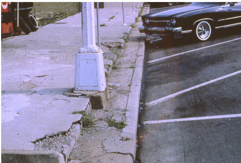
Figure 5. "Before the Public Improvement Project, streets and sidewalks were crumbling and dangerous." 53
