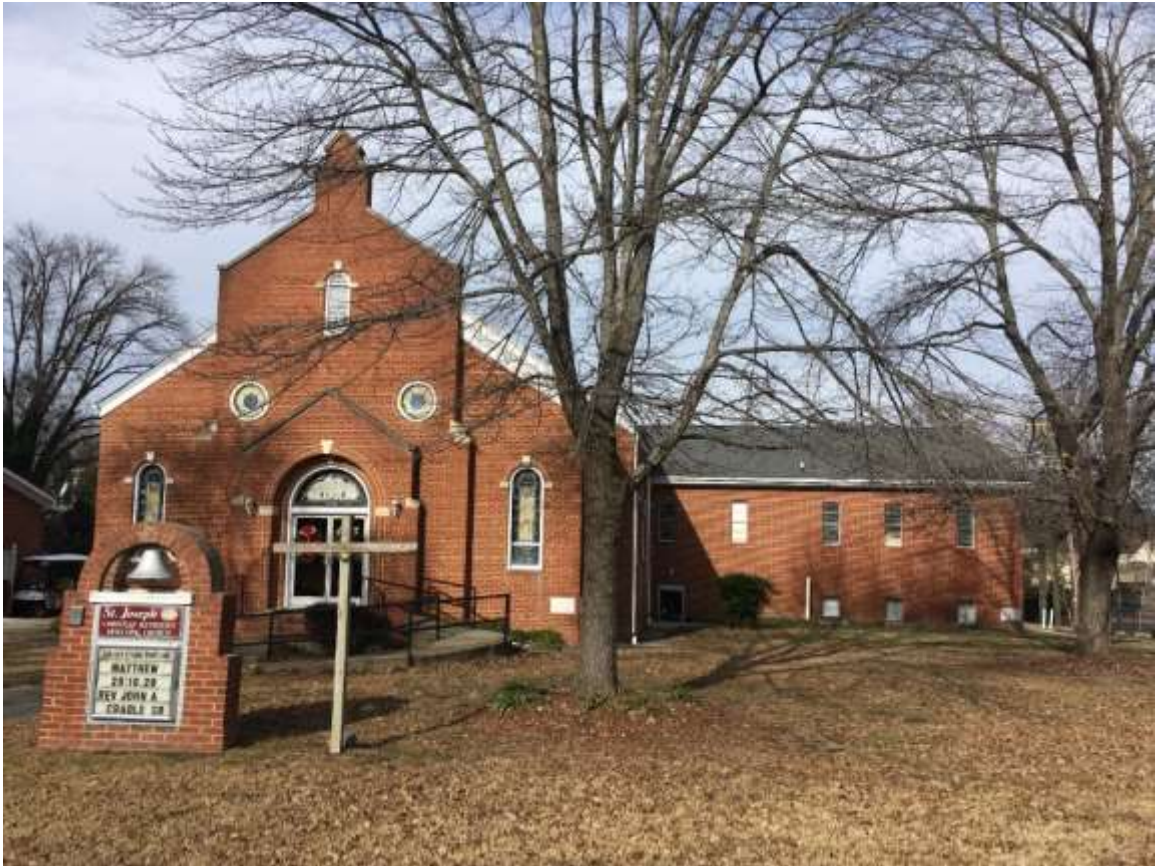
Figure 15. Front façade of St. Joseph CME Church
