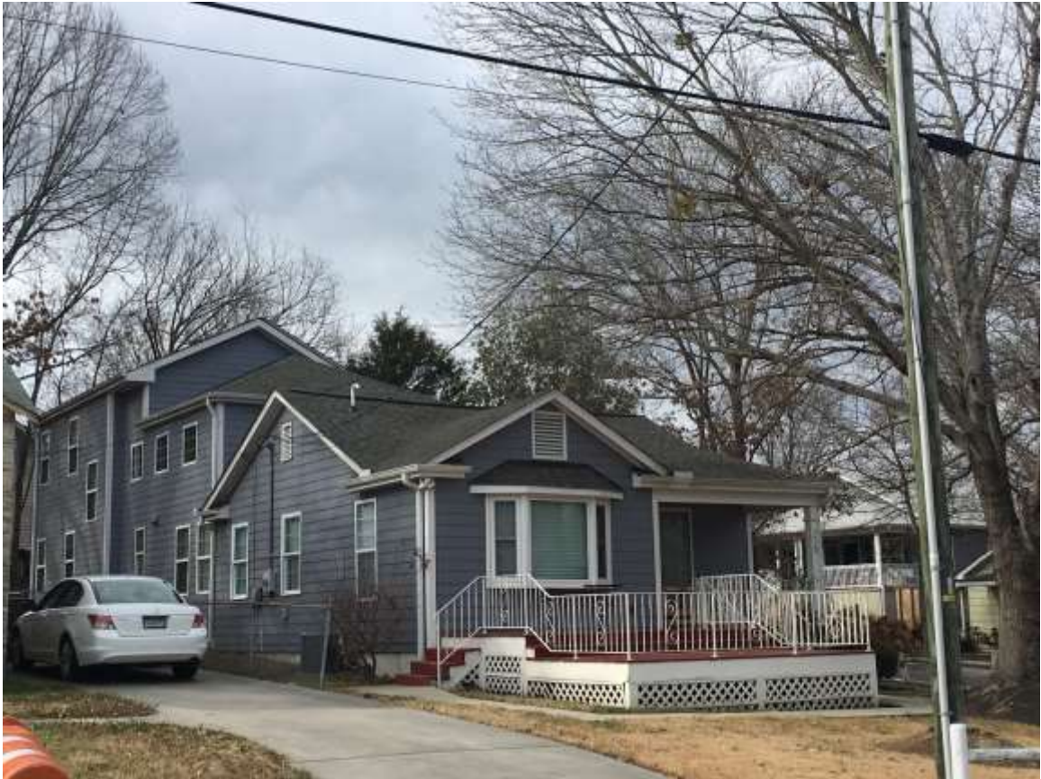
Figure 5. 229 Roberson Street west elevation showing rear addition
