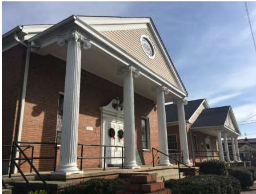
Figure 14. Front façade of First Baptist Church
