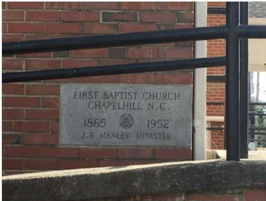
Figure 13. Cornerstone laid on north elevation of First Baptist Church
