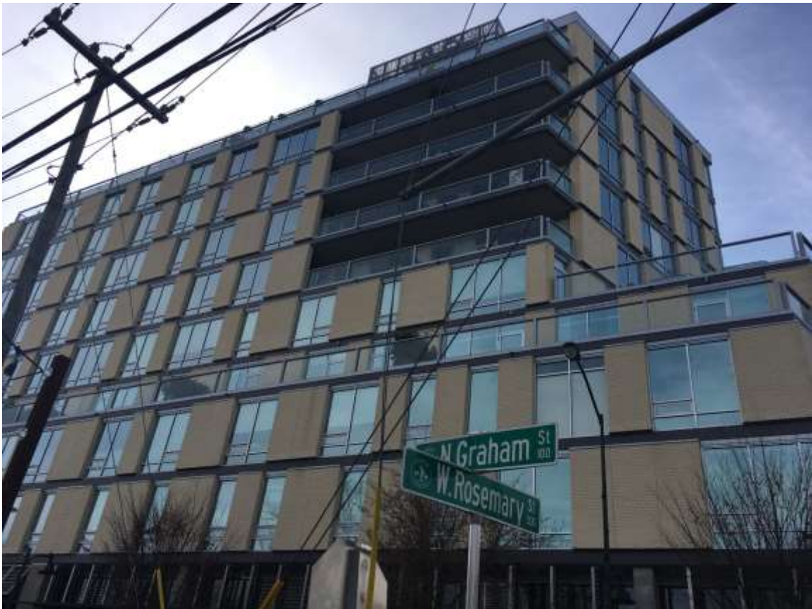
Figure 1. Image of Greenbridge Condominiums
