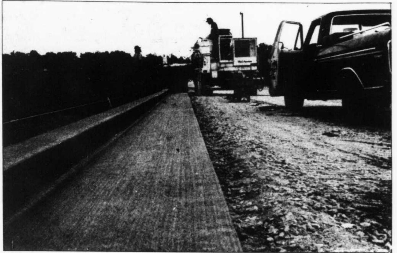
Workers put the finishing touches on MTSU Drive. The new street will connect the campus with Northfield Loop, which is also under construction.
