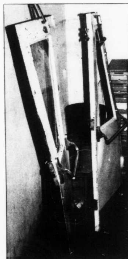
Cope Administration Building was just one of the several buildings on campus that sustained damage from the flood.
