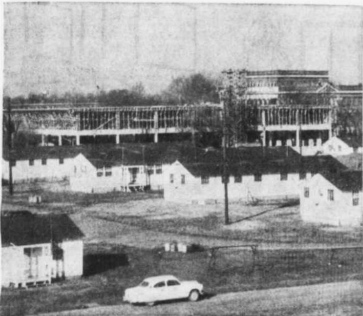
This unusual shot of the construction on the new library is made from the Fire School observation tower looking west by Jim Keathley of the News Journal. The Veteran's apartments are in the foreground and the administration building peeps demurely from behind the construction. In the center background can be seen the top of the Union building.
