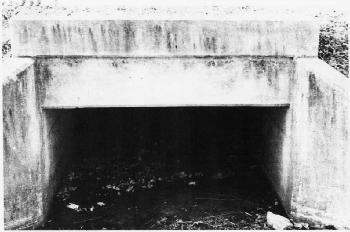
This ditch is one of many drainage problems on the MTSU campus. The school has joined forces with Rutherford County and the City of Murfreesboro in an effort to correct the situation.
