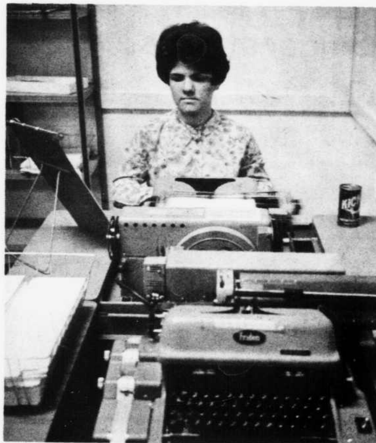
Miss Rosalind Elston, production supervisor for the SIDELINES, makes a special tape of all stories that are to be published. This coded tape is then fed into a reproducing machine that prepares justified columns.
