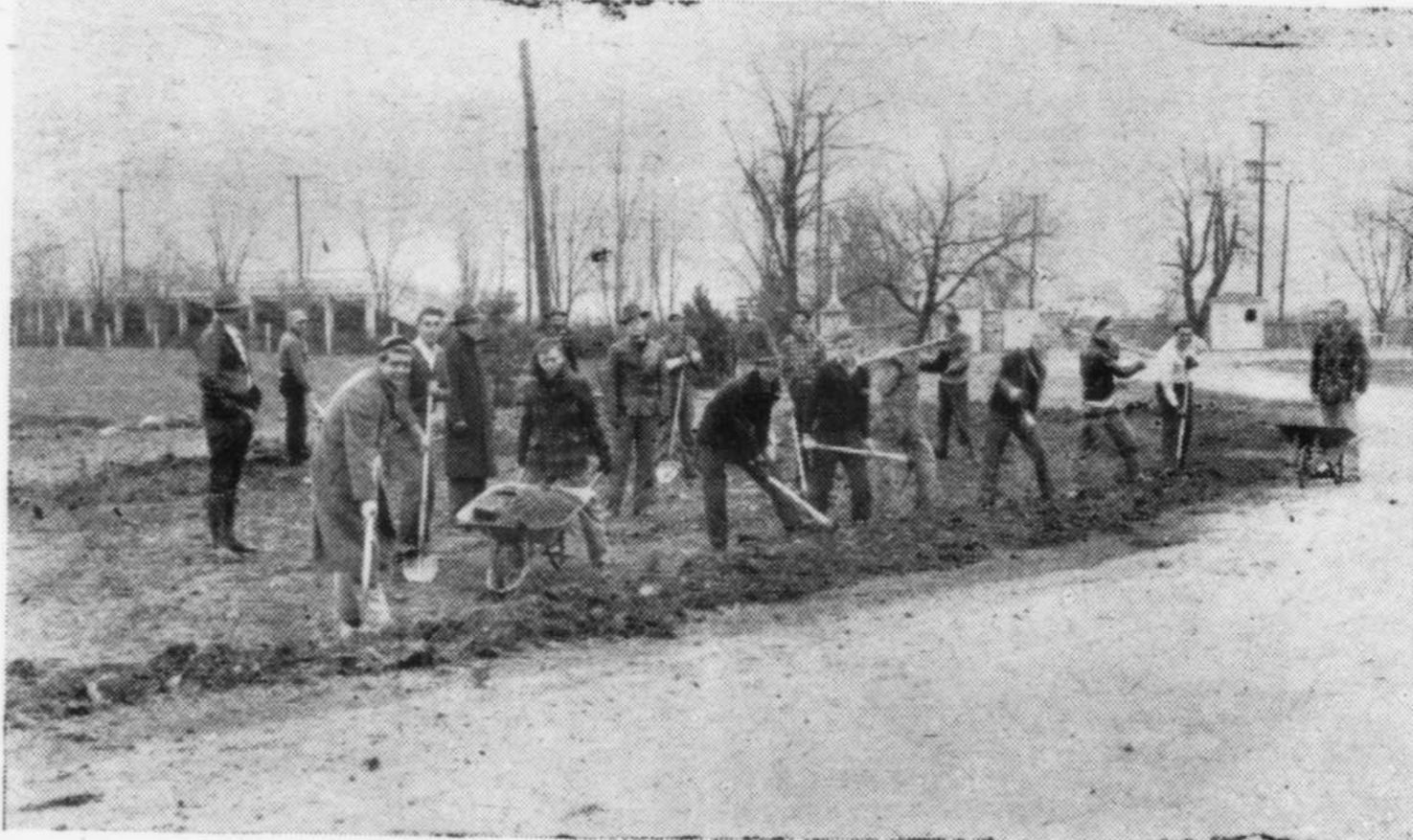
Shown above is a group of NYA workers as they began breaking ground on the site of the new $15,000 NYA work building which will be located on the main drive just behind the Administration and between the cafeteria and power house. Work is under the direction of Leon Bibb and W. A. Mays and will consist entirely of NYA help. The building should be finished by next spring.
