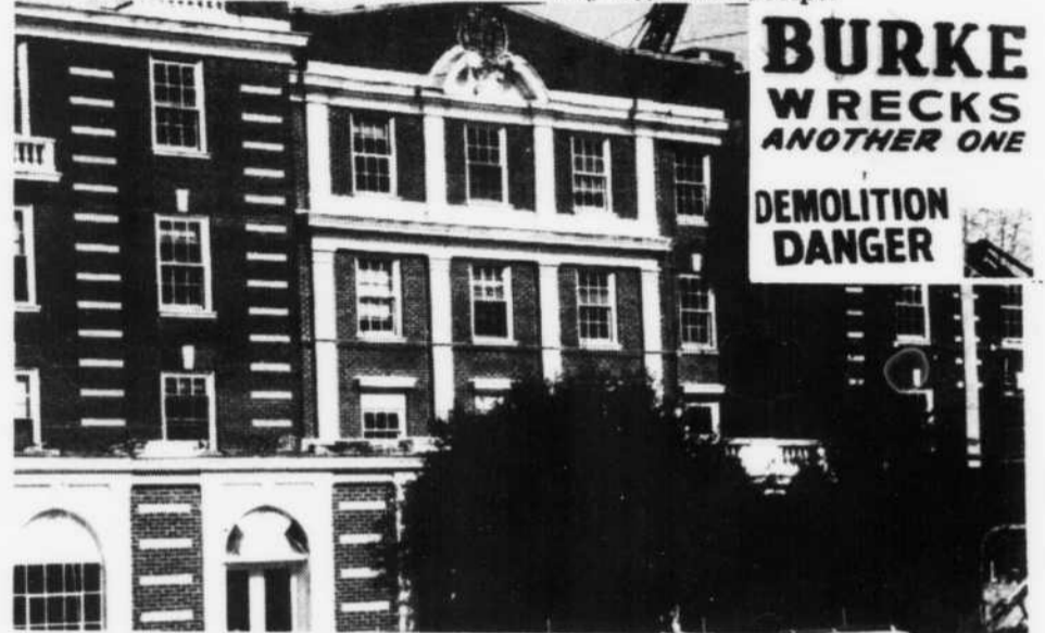
Demolition of Murfreesboro's historic James K. Polk Hotel began Thursday and will continue for the next 30-60 days to make way for a new, modern bank building. Staff photo by Thom Coombes
