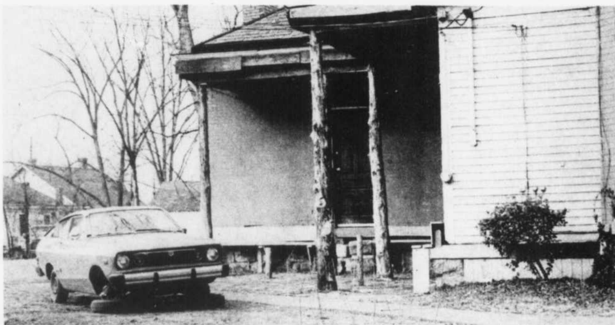
Sigma Chi's landlady claims that fraternity members have not made necessary repairs to the house they rent.
