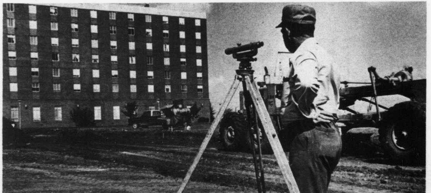
A construction worker surveys the sight of the tennis courts now under construction near Cummings Hall.
