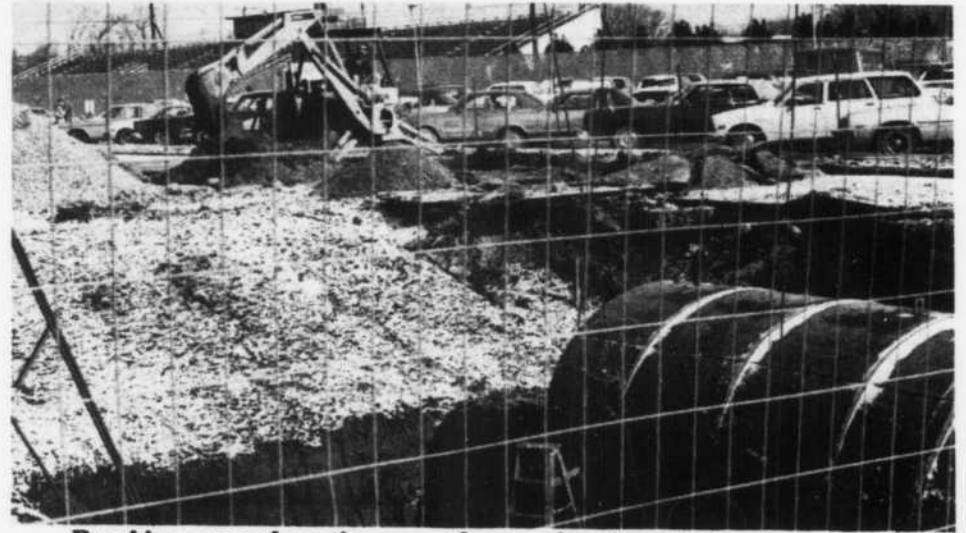
Breaking ground continues on the new heating plant to be located behind Old Main. Completion of the building is expected in July, 1978.
