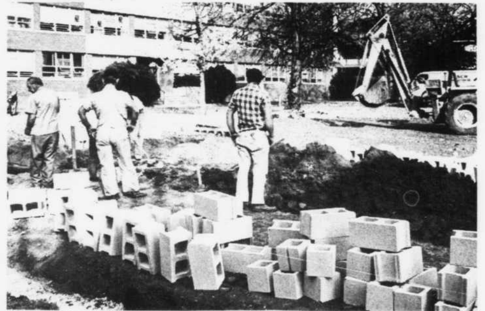
With an expected completion date of early next year for the laundromat being built between Sims and Beasley halls, workmen are busy working while the weather holds. [Robin Rudd photo]
