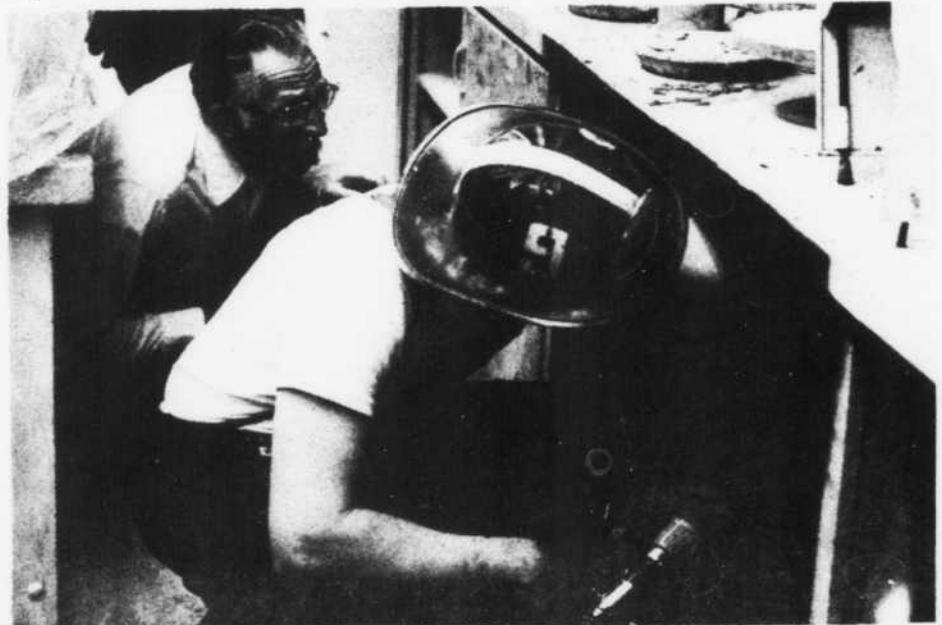
Archie Sullivan, MTSU safety director, and Jerry Goodman Murfreesboro fire captain, inspect damage resulting from Tuesday morning's fire at the Art Barn. The cause of the fire was unknown. [Thom Coombes photo].
