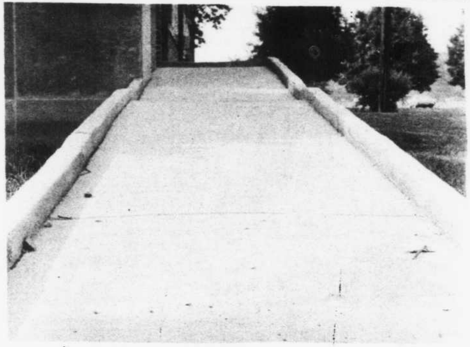
This ramp leading up to the music building was recently installed to aid handicapped students. [Debra Ross photo]
