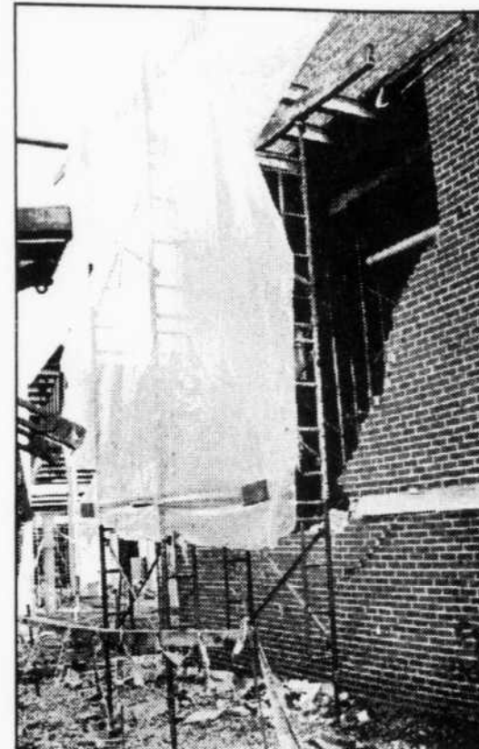
Jason Mazzo/staff On Tuesday, October 28, a crane knocked a 15- by 20-foot hole in the north wall of the natatorium. The crane was being used on the new football stadium press box.
