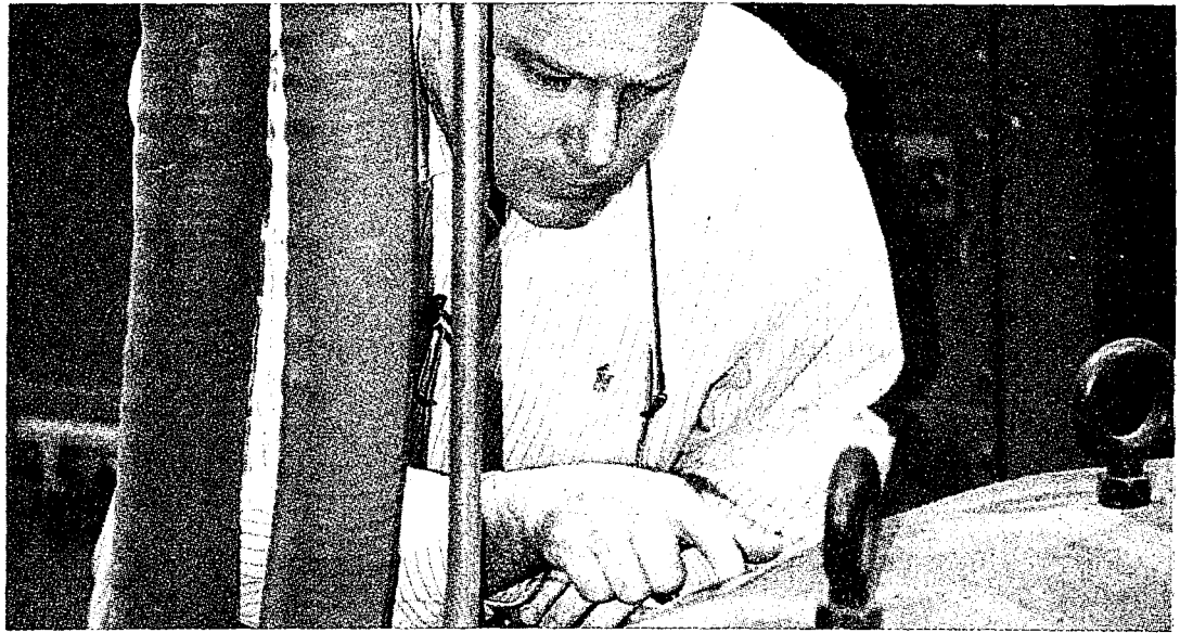
Photo by Jay Bailey, photography editor Joe Whitefield, executive director of Facilities Services Department and director of the Center for Energy Efficient, gives a tour of MTSU's Central Utility Plant on campus earlier this semester.
