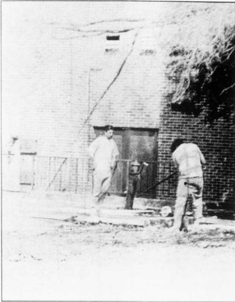
Vickie Gibson/Staff These facility services employees continue drainage maintenance work on Corlew Residence Hall.
