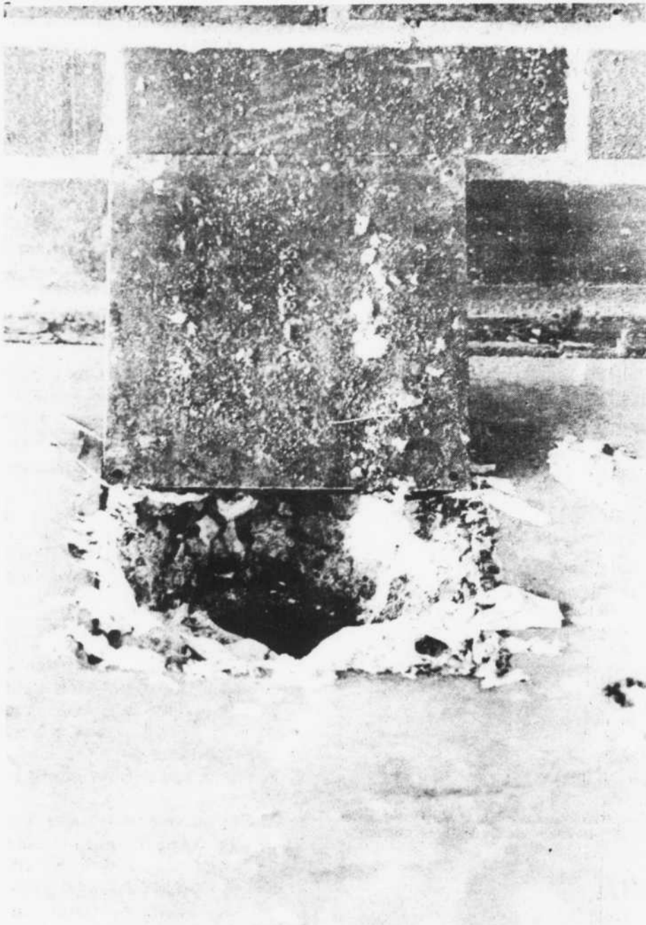
Human wastes and other sewage often back up this excess pipe in the breezeway of married housing's "G" complex. The pipe has been left open to counteract sewage overflows that could flood residents' homes. Charles Steed photo
