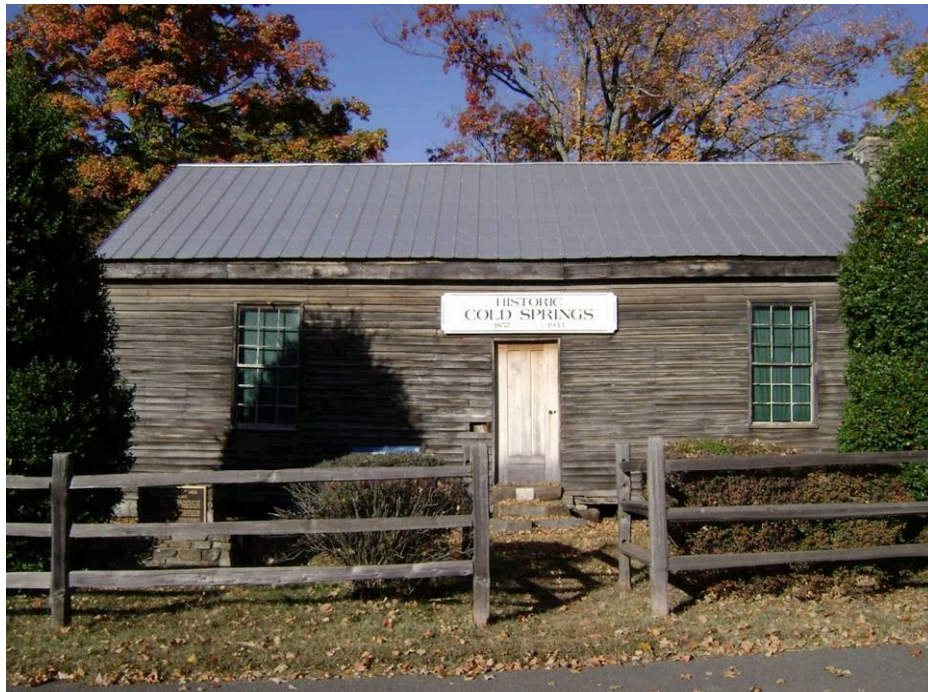
Figure 16. Cold Spring School constructed ca. 1857. Courtesy TCWNHA, 2010.
