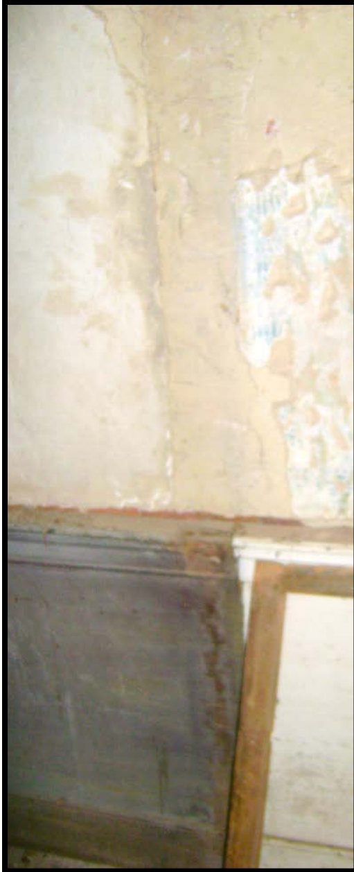
Figure 3.21. Partition wall ghost marks. (Jessi White)
