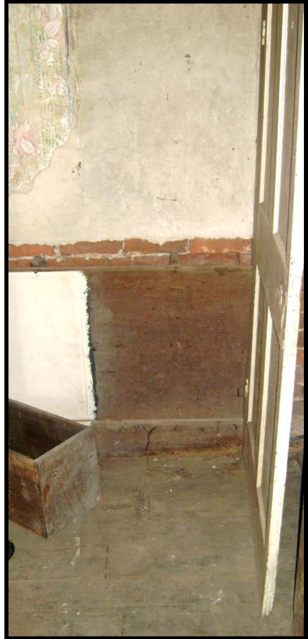
Figure 3.22. Partition wall ghost marks. (Jessi White)
