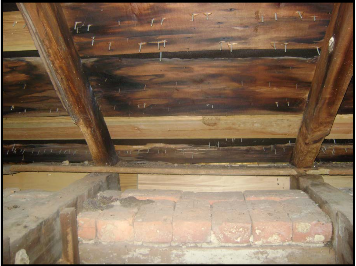
Figure 3.17. False plate, ceiling joists, and rafters, Hawthorn Hill. (Jessi White)
