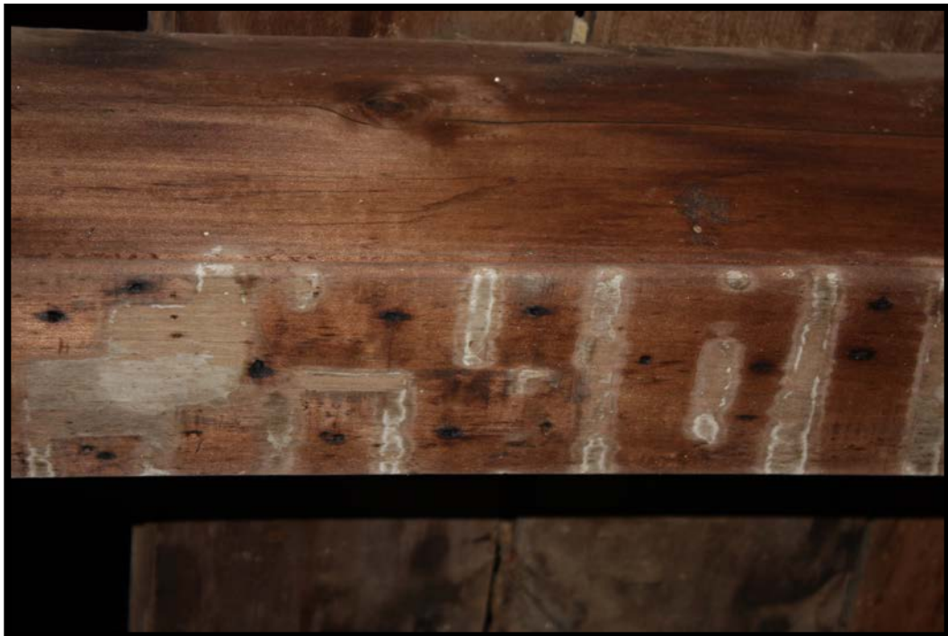
Figure 3.6. Second story joist with bead, Hawthorn Hill. (Jessi White)
