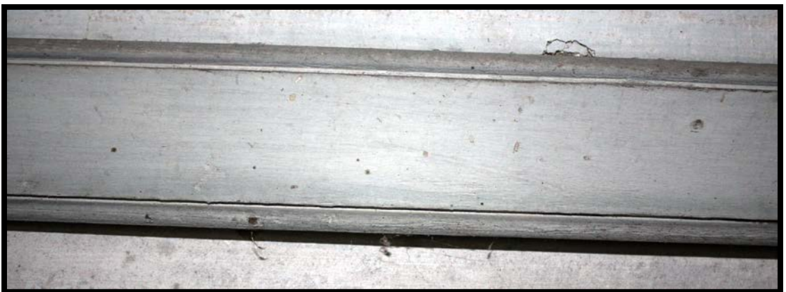
Figure 3.14. Second floor chair rail, Hawthorn Hill. (Jessi White)
