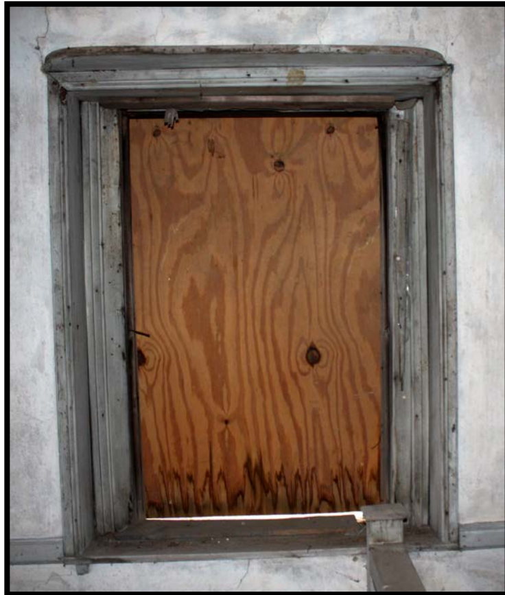
Figure 3.11. Second floor window molding and apron, Hawthorn Hill. (Jessi White)
