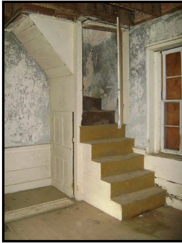
Figure 3.31. Boxed winding staircase, parlor. (Jessi White)
