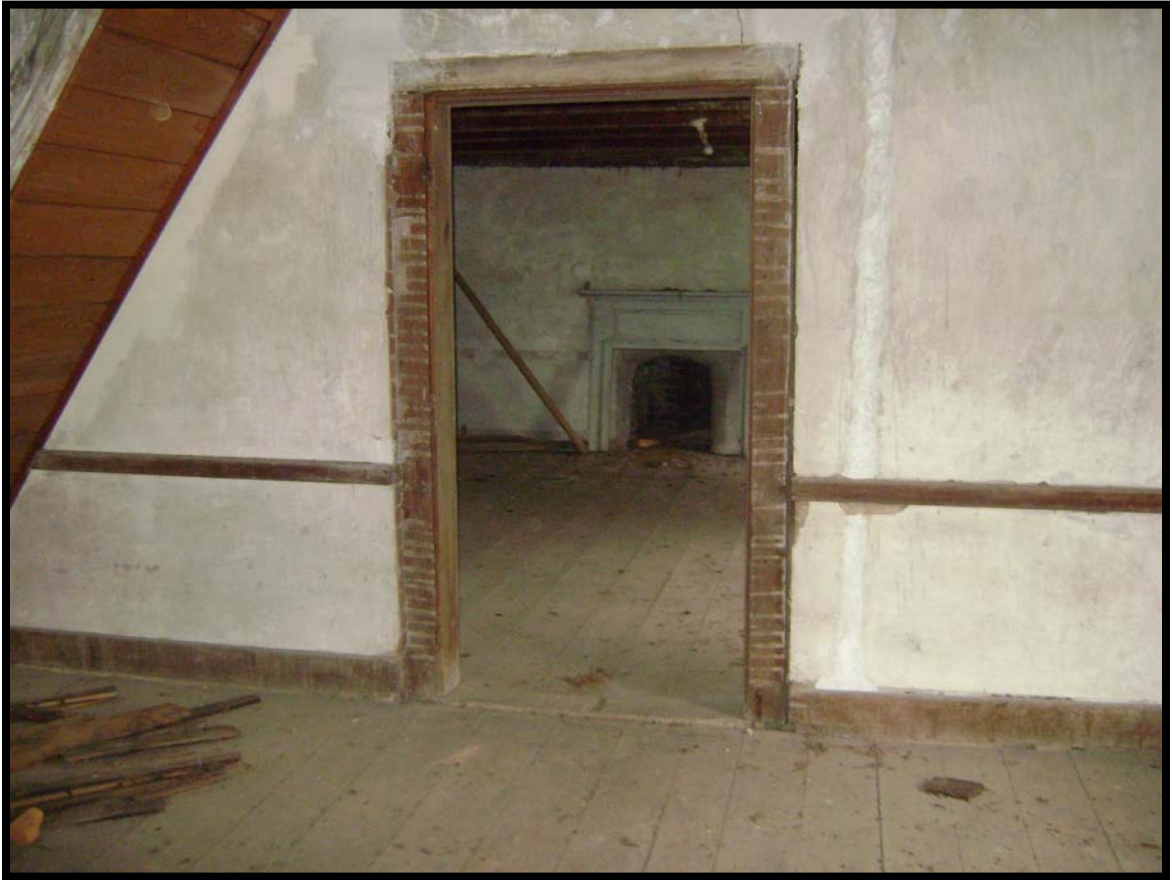
Figure 3.30. Interior second story doorway with lath and plaster ghost marks (Jessi White)
