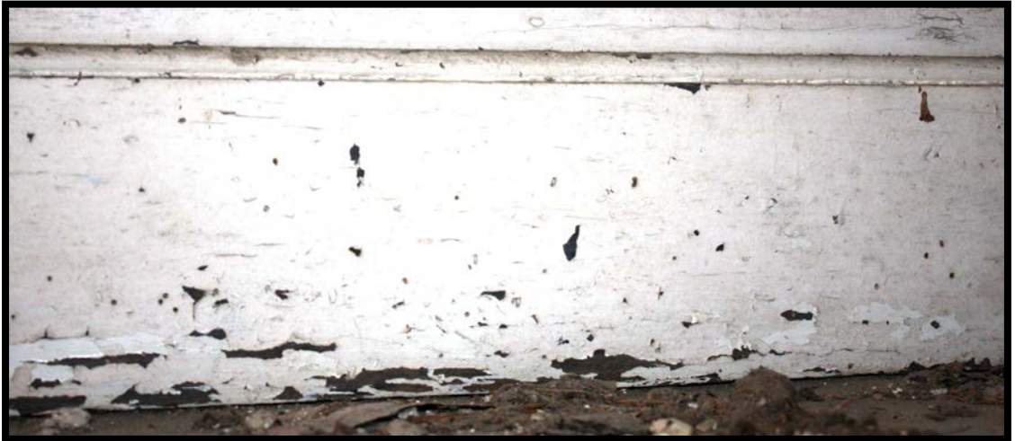
Figure 3.13. First floor baseboard, Hawthorn Hill. (Jessi White)
