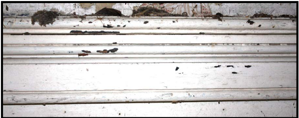
Figure 3.12. First floor chair rail, Hawthorn Hill. (Jessi White)
