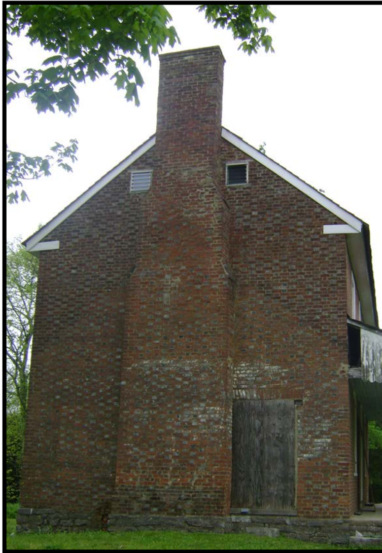
Figure 3.9. West wall chimney, Hawthorn Hill. (Jessi White)
