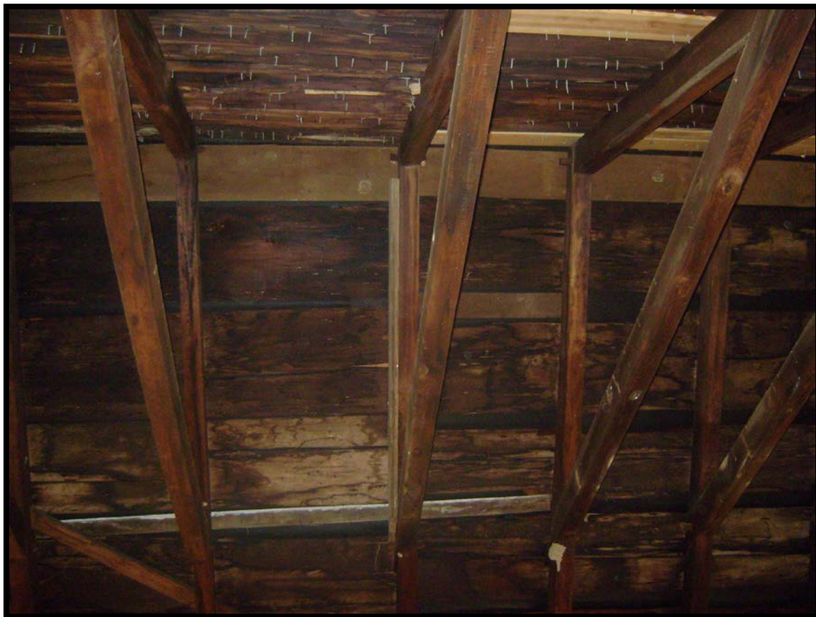
Figure 3.16. Lap-and-peg joinery and collar ties, Hawthorn Hill. (Jessi White)
