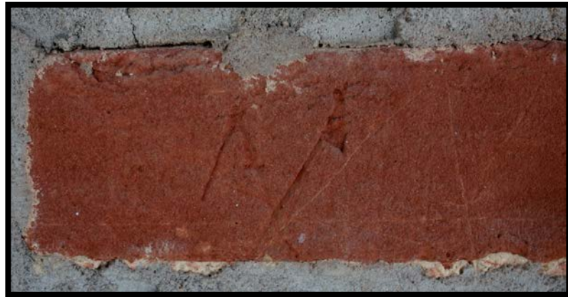
Figure 3.7. Maker's mark on brick work "M", Hawthorn Hill. (Jessi White)
