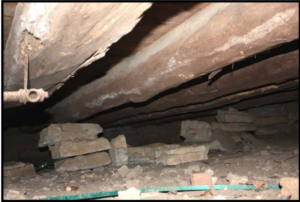
Figure 3.5. Log sleeper joists and limestone supports, Hawthorn Hill. (Jessi White)
