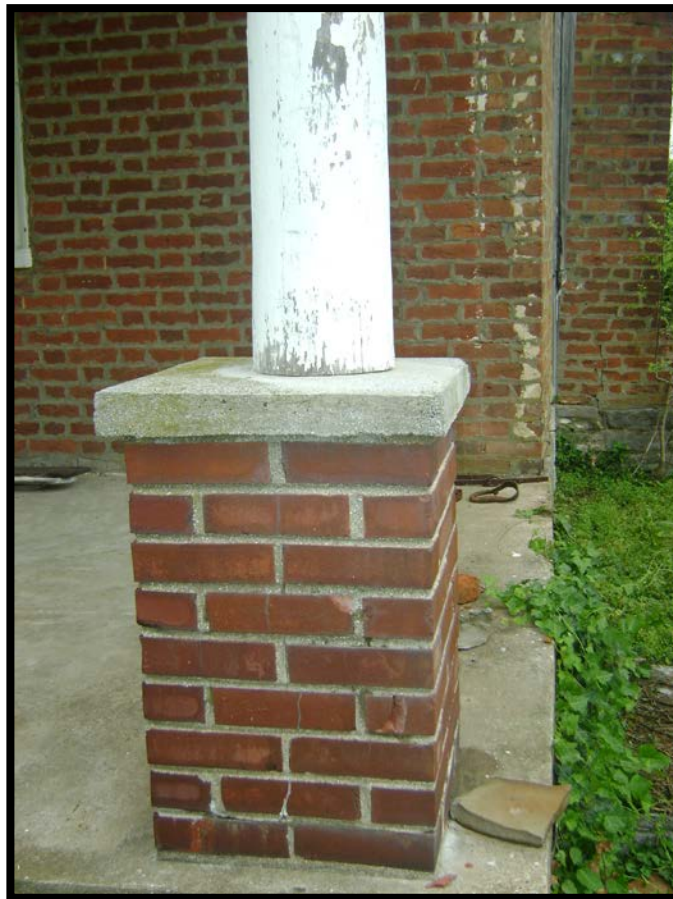
Figure 3.45. Brick column base and concrete pad added, circa 1960 to Hawthorn Hill. (Jessi White)
