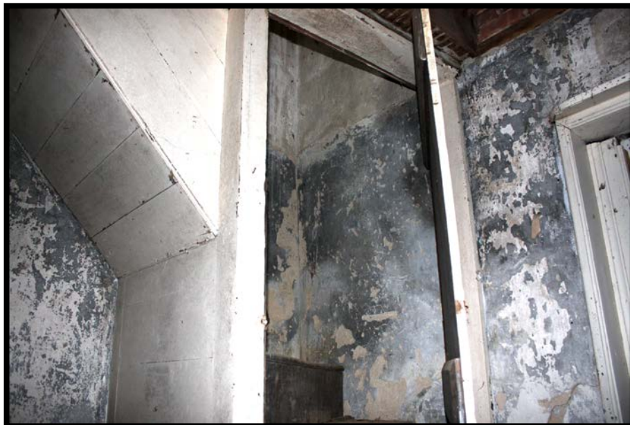
Figure 3.32. Interior view of boxed stair showing paint line where the stair was cut in. (Jessi White)
