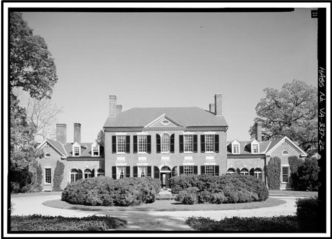
Figure 2.9. Woodlawn, 9000 Richmond Highway, Mount Vernon, Fairfax County, VA. (HABS image)
