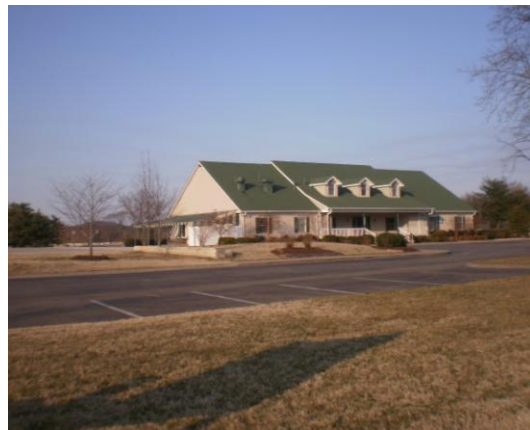
Fig. 31 The former Country Club Clubhouse and parking lot. The sign for the Eastern Flank Battlefield Park is to the left of the photo as is the Civil War Trails marker. Photograph courtesy of Rachael Finch, October 2010.
