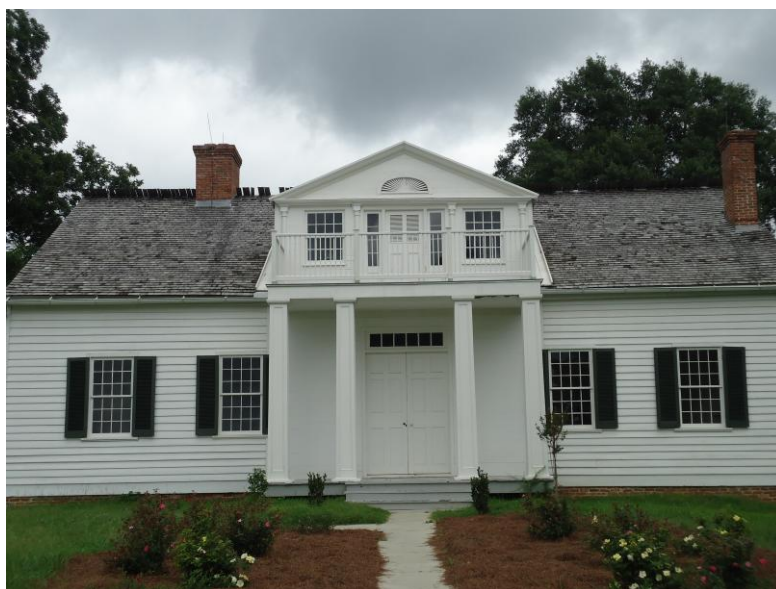
Fig 23 The Shirley house completely stabilized, it meets ADA standards, with an elevator and parking in the back. Newly installed concrete pathways and handrails are additions too. February, 2013.
