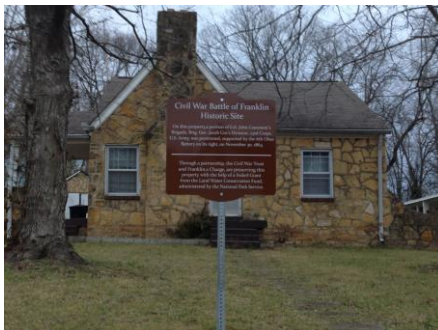
Fig 36 This home will be relocated to another part of Franklin or Williamson County and the lot will serve as part of the upcoming Carter's Cotton Gin site. The site is in partnership with the Civil War Trust. March 3, 2013
