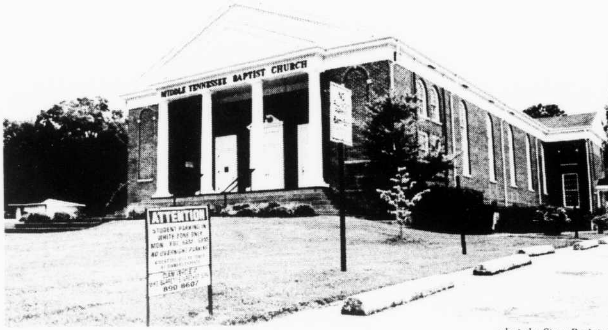
The new Middle Tennessee Baptist Church on Tennessee Blvd. is enforcing strict parking rules.
