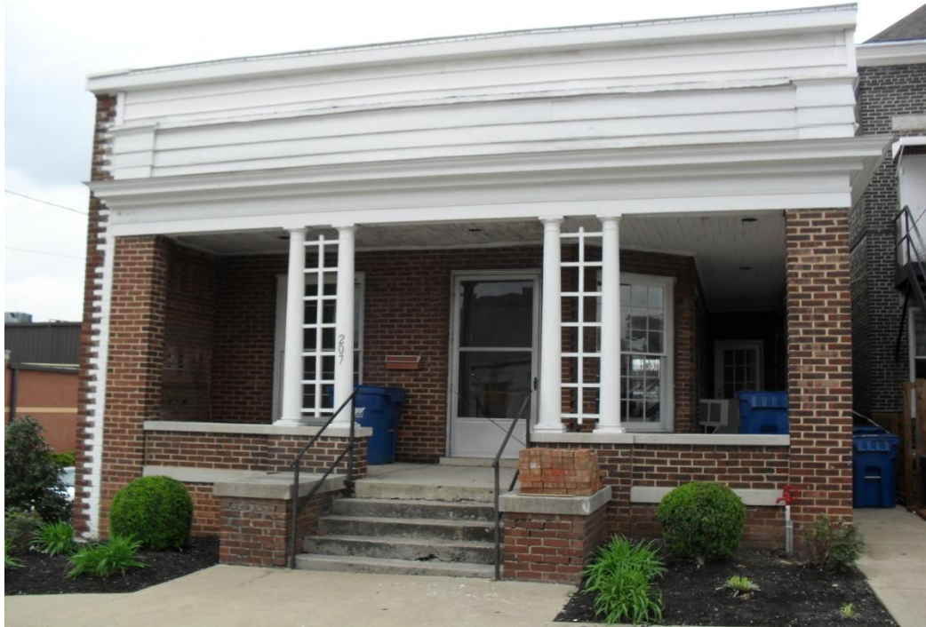
Figure 6.1 West elevation, Lewisburg Ladies Rest Room, image by author, April 2011.
