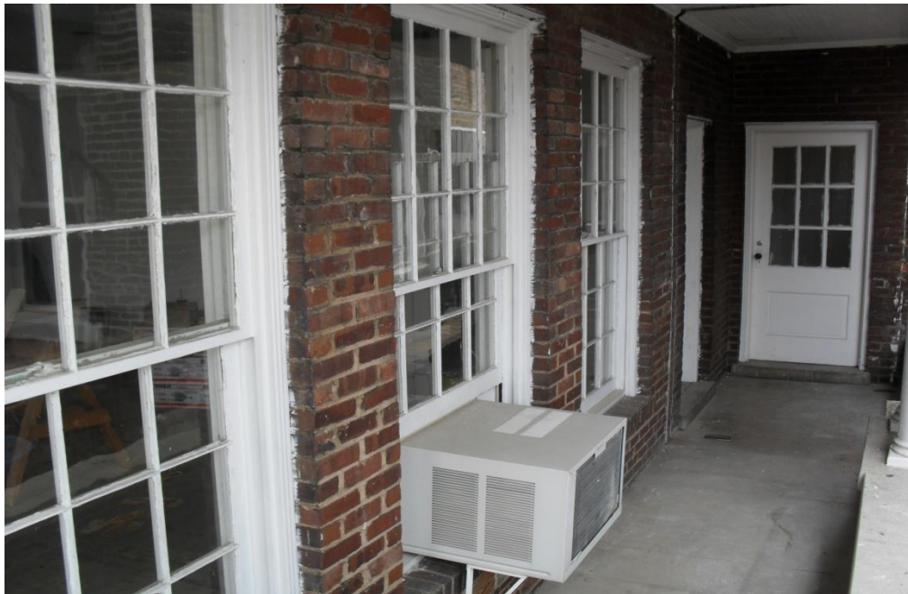
Figure 6.3 South elevation porch, showing doors to alcove and former kitchen, Lewisburg Ladies Rest Room, image by author, April 2011.
