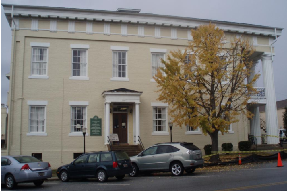
Figure 4.3 South exterior elevation, Main Street entrance, Newberry Ladies Rest Room, image by author, December, 2011.
