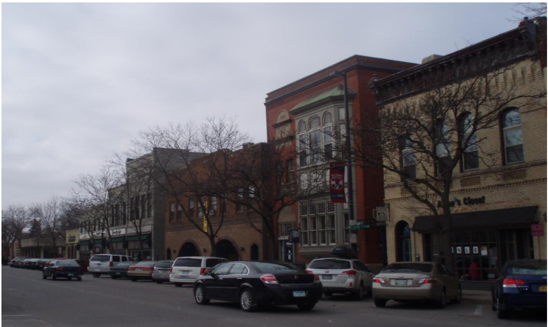
Figure 5.5 Façade of the current Northfield Arts Guild Building (second from right), former Northfield Community Hall, located in the Northfield central business district, image by author, February 2012.
