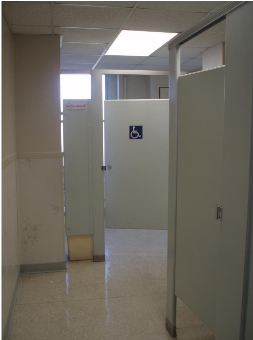
Figure 2.5 Facing East, location of current and historic ladies toilet facilities, Rice County Courthouse, image by author, January 2012. The dropped ceiling and fluorescent lighting likely date to renovations that occurred c.1983.
