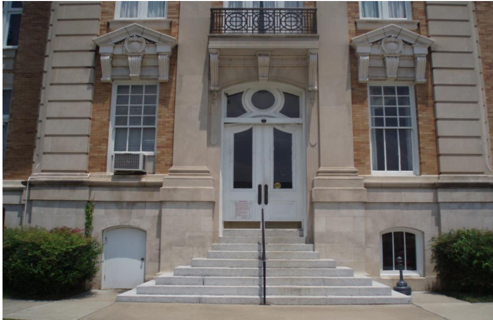
Figure 3.4 Original exterior entrance to Pulaski Ladies Rest Room, South elevation, image by author, July 2011.
