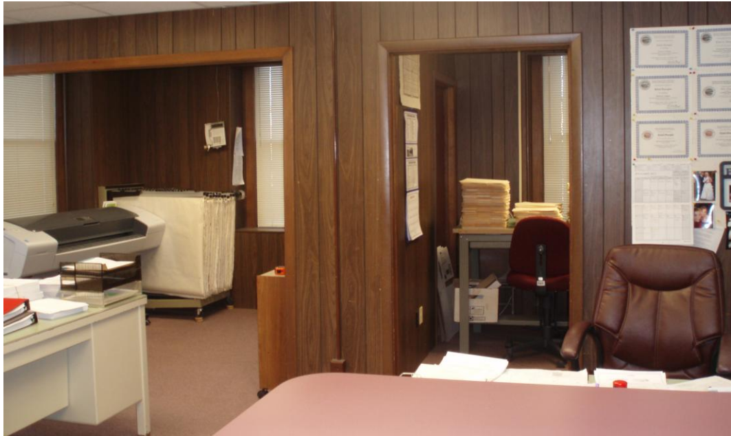
Figure 2.6 Northeast elevation, historic location of lounge area of Lyons Ladies Rest Room, Rice County Courthouse, image by author, January 2012. It is likely that the interior partitions and faux wood paneling were added in renovations that occurred c. 1983.
