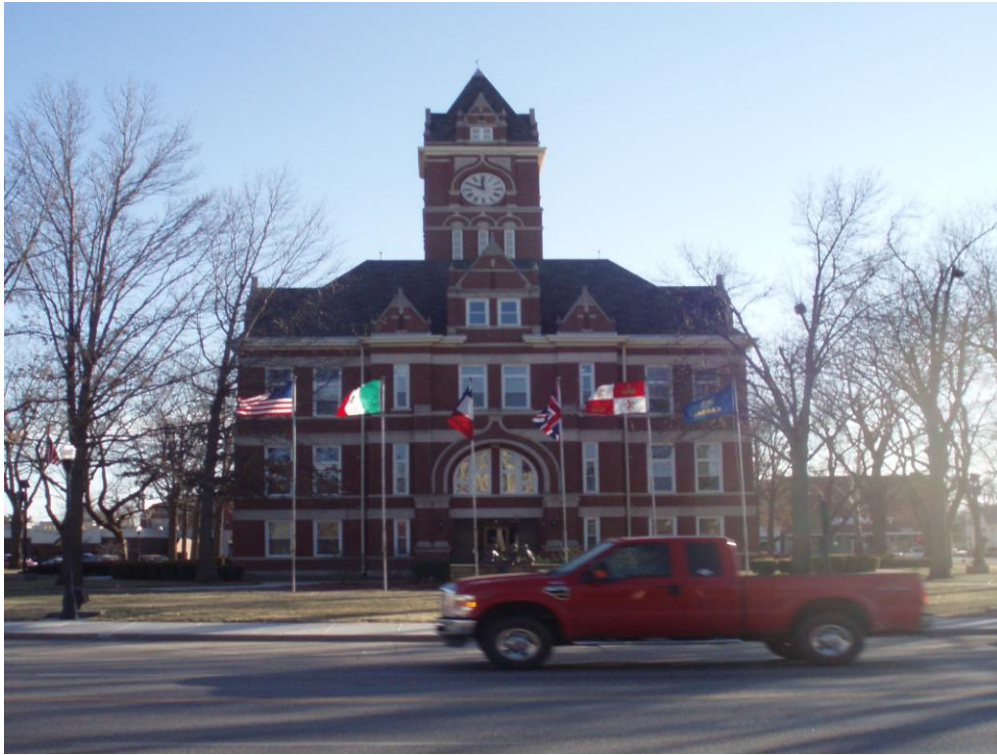
Figure 2.2 North elevation, current Rice County Courthouse, constructed and dedicated in 1911, image by author, January, 2012.
