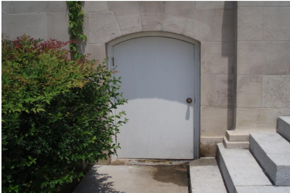
Figure 3.5 Original exterior entrance to Pulaski Ladies Rest Room, South elevation, image by author, July 2011.
