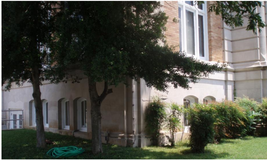
Figure 3.8 Exterior Southwest elevation, showing ladies rest room area, image by author, July 2011.
