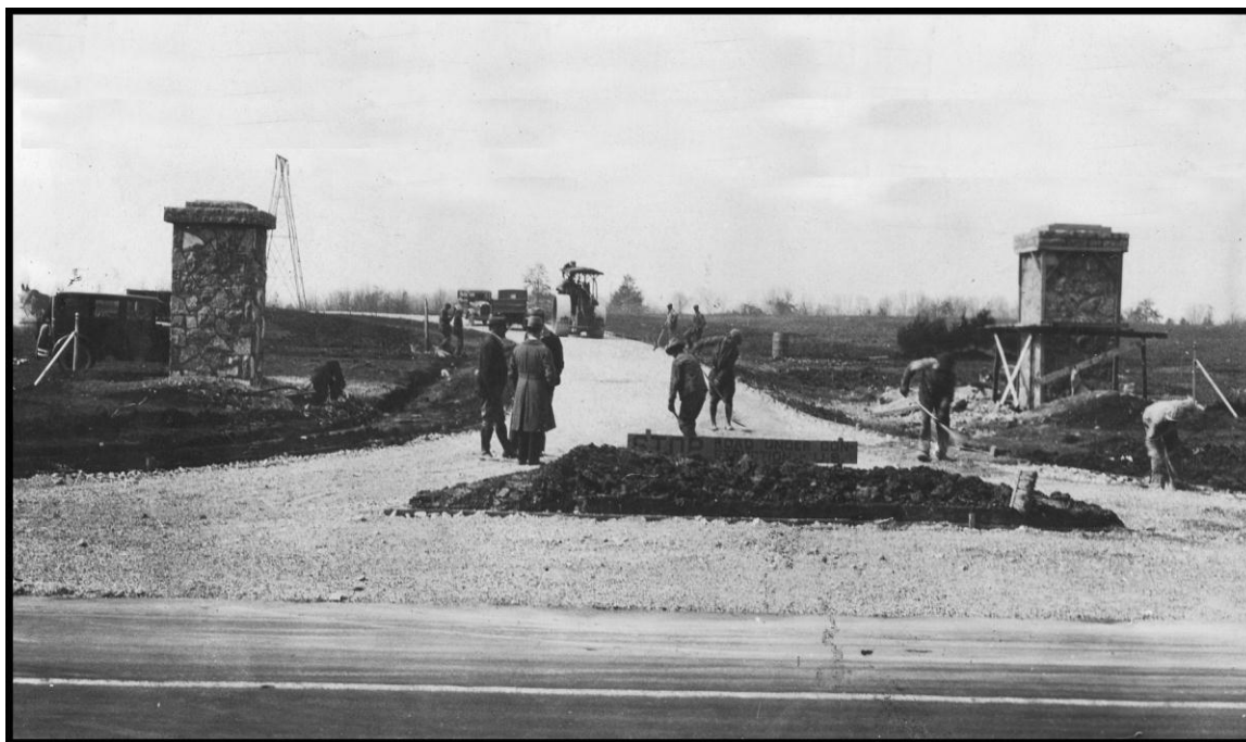
Figure 21. Stone Columns at the North Entrance. These columns were built by Herbert Smith in 1931. In this image, the cannonball pyramids that would top the columns have not yet been placed. Stones River National Battlefield.
