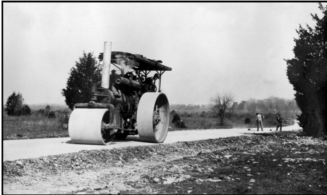
Figure 20. Park Road Construction. Conner included this photograph in a 1931 progress report to the Quartermaster General's office. Stones River National Battlefield.
