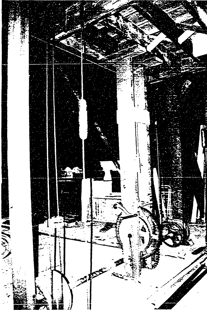
Figure 5.28 Second-story left to raise carriages from the first floor room to the storage area in the Coach Barn (1901), Shelburne Farms, Shelburne, Vermont. July 2003.
