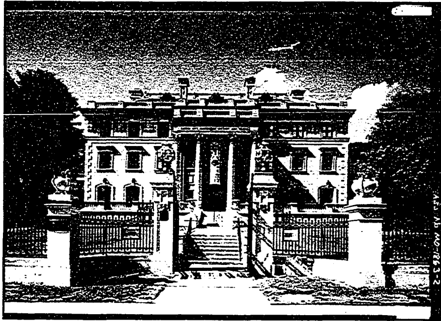
Figure 5.39 Corinthian Hall (1910), Kansas City, Missouri. Courtesy of the Library of Congress, Prints and Photographs Division, Historic American Buildings Survey, HABS.MO-1863-2.
