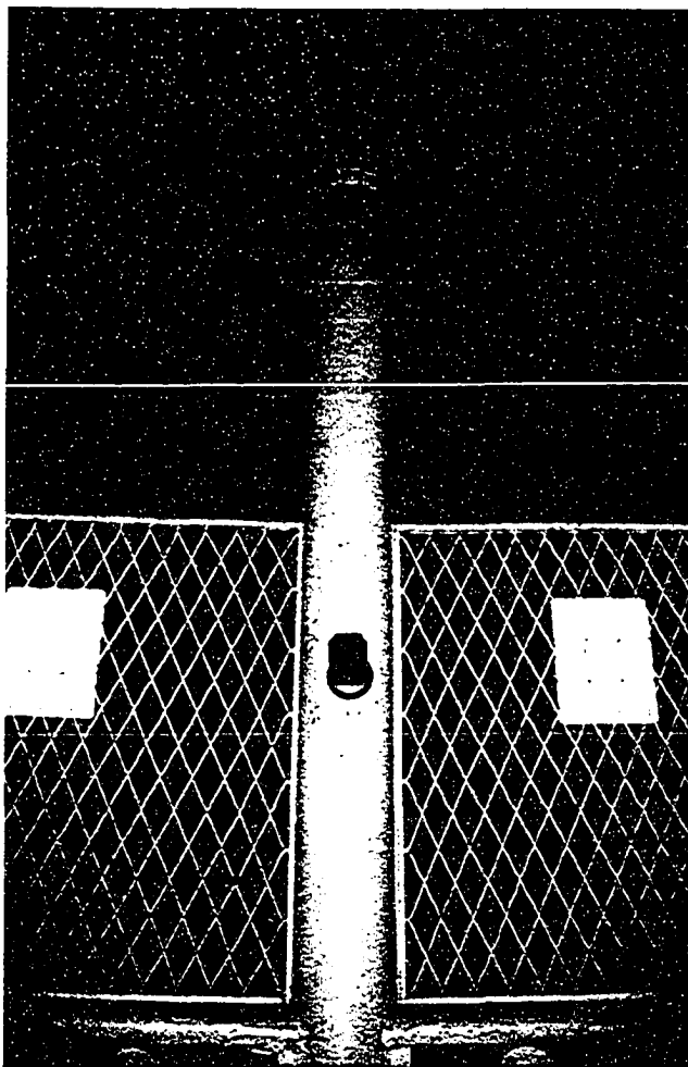
Figure 4.6 Aisle tie ring on fancy support post and metal stall fronts in the Roosevelt Stable (1886), Hyde Park, New York. July 2002.
