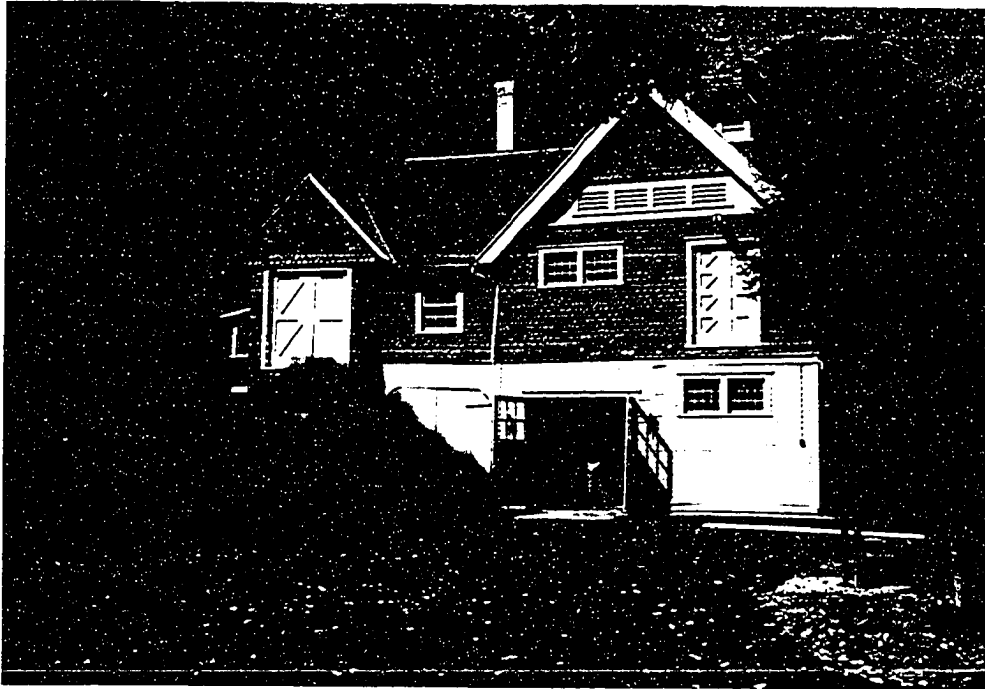
Figure 6.8 Exterior of the Roosevelt Coach House-Stable (1886). FDR/Vanderbilt National Historic Site. Nancy A. Morgan Photograph. September 2004.
