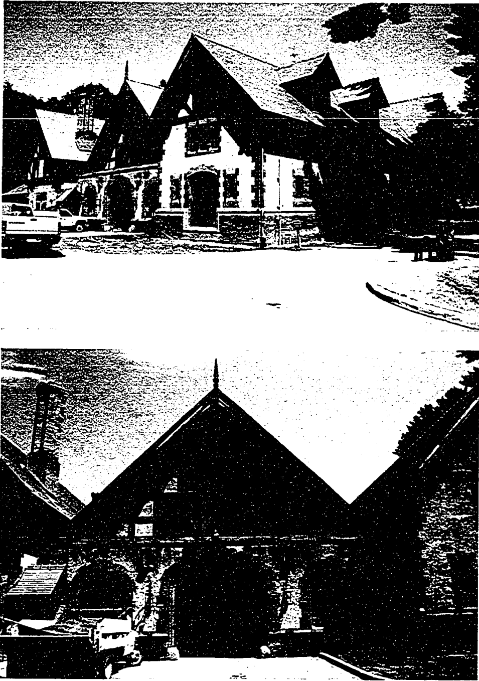
Figure 6.1 Coach house and garage (1897) at Vanderbilt Mansion, Hyde Park, New York. July 2002: top, side view; bottom, main entrance.
