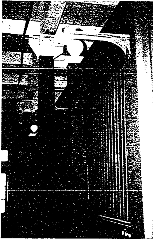
Figure 5.80 Box stall front, side view, with blanket bar and halter hook in the Show Horse Barn (1914) at Longview Farm, Lee's Summit, Missouri. March 2004.
