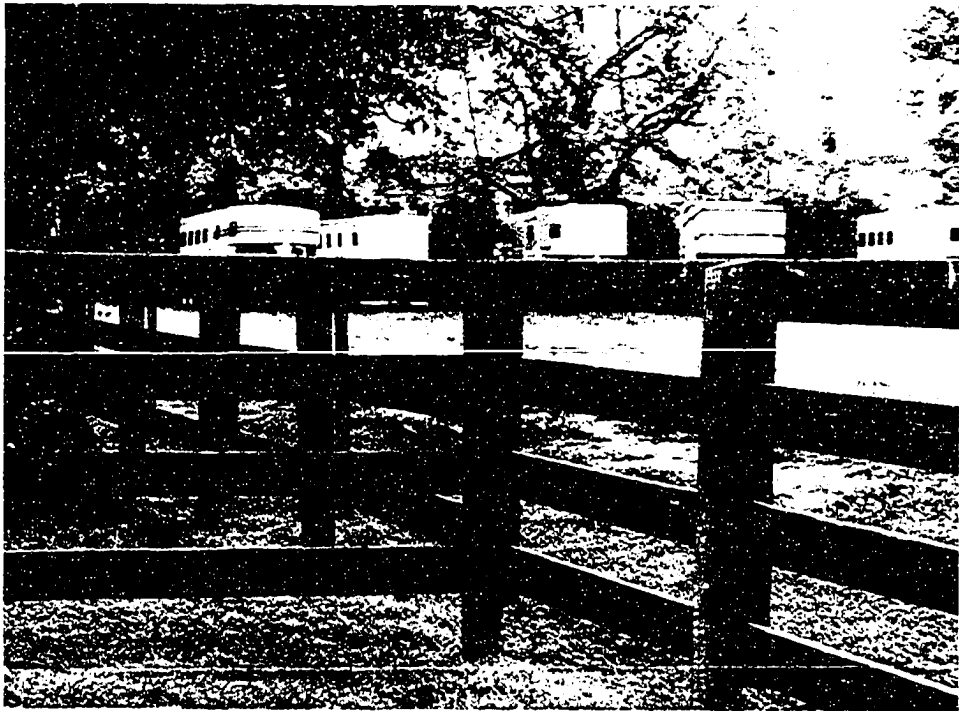
Figure 4.49 Board fencing showing protective facing boards in corner. Brownland Farm, Franklin, Tennessee.
