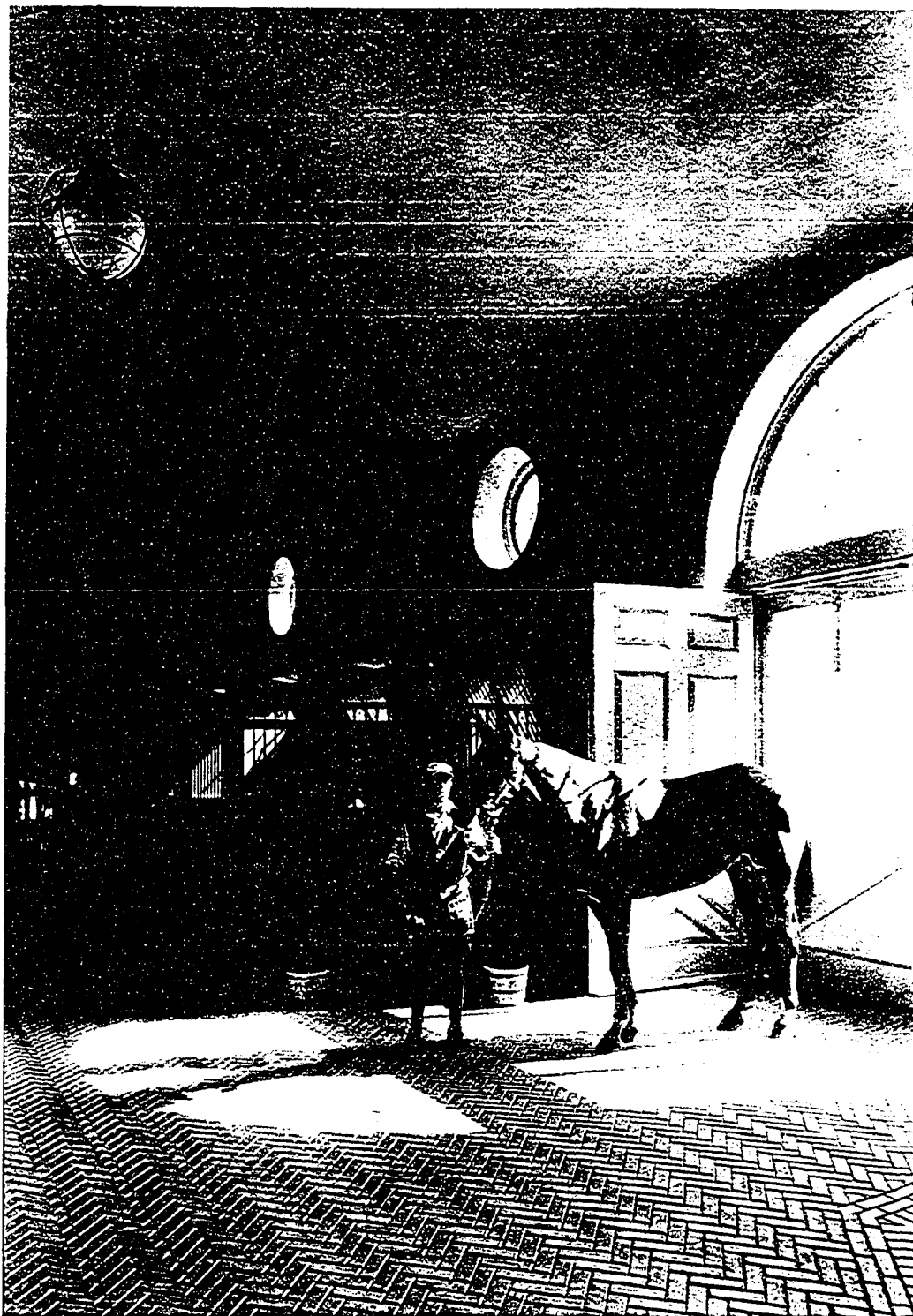
Figure 4.85 Polo stable at Caumsett, Long Island with high ceilings and windows, brick aisle, water buckets, and overhead radiators. Samuel H. Gottscho Photograph. 12 October 1933. Courtesy of the Library of Congress, Prints and Photographs Division, Gottscho-Schleisner Collection, LC-G612-20793.
