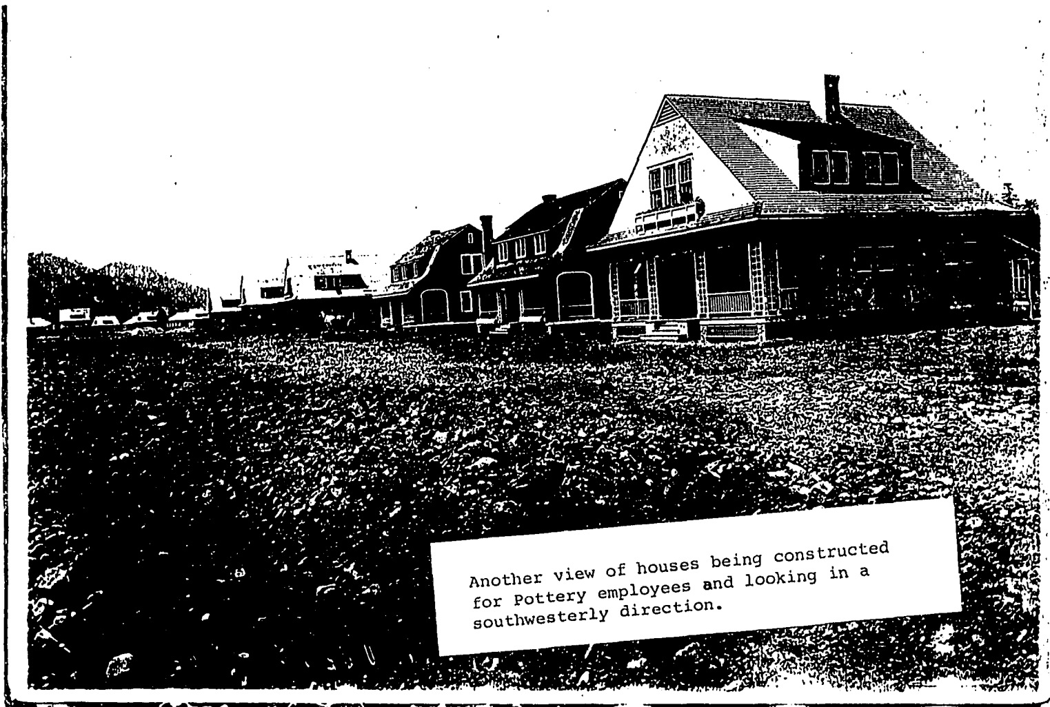
Figure 29. A Closer View of Houses under Construction
