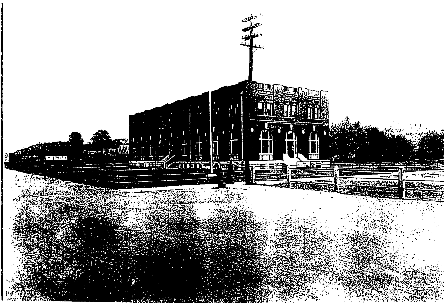
Figure 17. CC&O General Office Building
