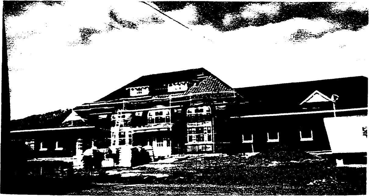
Figure 59. Clinchfield Depot, during renovation
