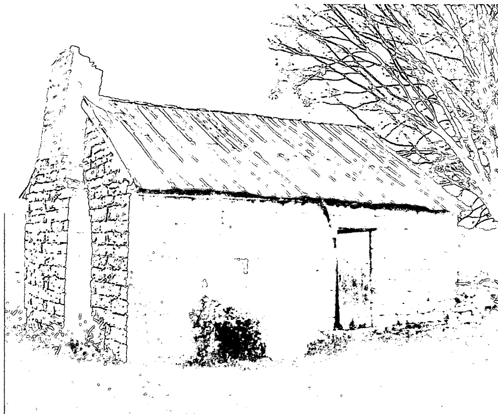
Figure 4.3 Crenshaw farm slave house, the only stone building recorded by the survey. Hartsville vicinity, Trousdale County.
