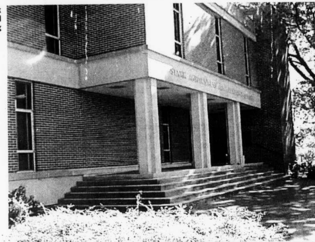
Stark Agricultural Building
