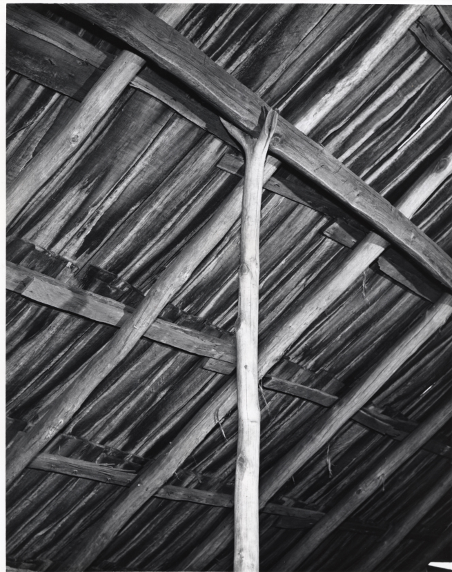
Figure 20. Interior of Willie Gibbons Barn. Photographed by Earl Palmer. Courtesy of Cumberland Gap NHP Archive.
