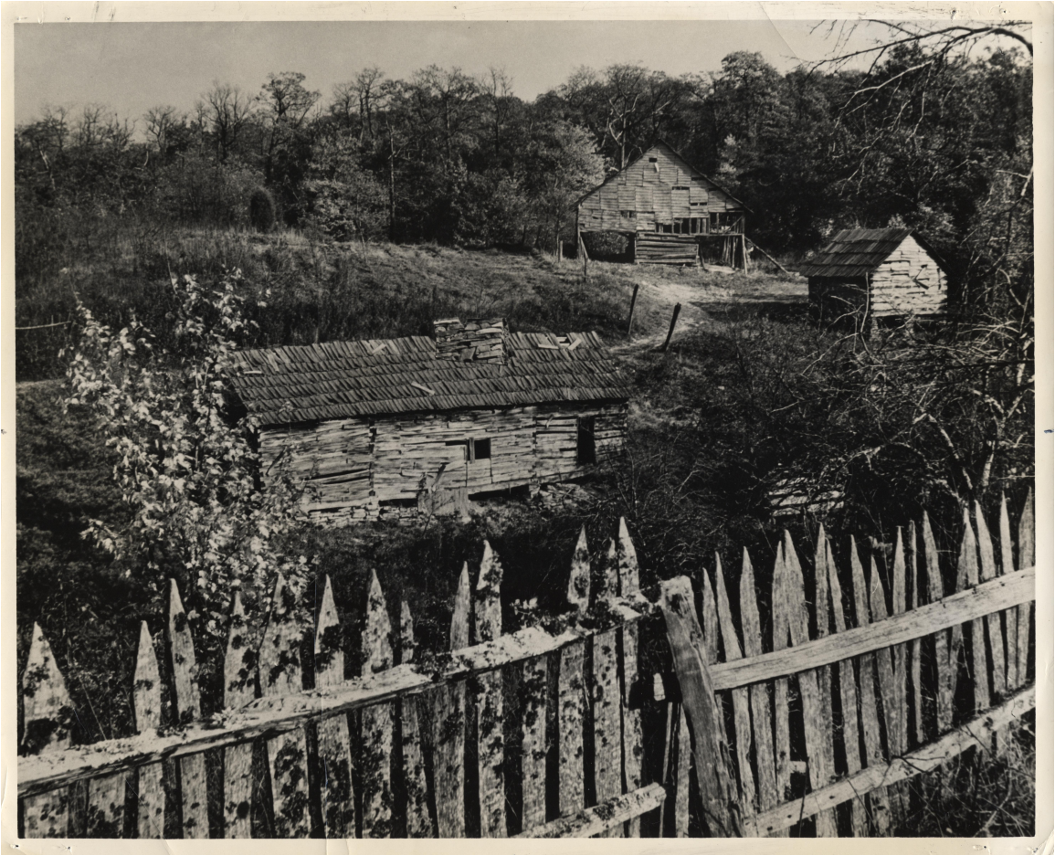
Figure 19. Willie Gibbons Farm. Photographed by Earl Palmer, October 17, 1965. Courtesy of Cumberland Gap NHP Archive.
