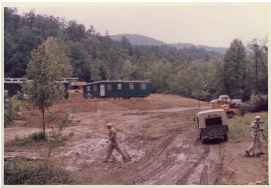
Figure 28. "Even in Mud, Work Goes On as Center Grows." Photographed in spring 1965. Courtesy of Cumberland Gap NHP Archive.
