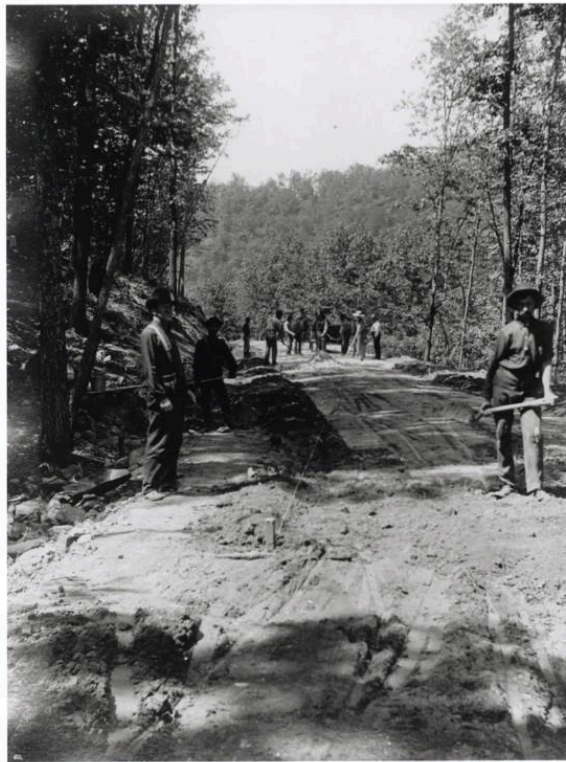
Figure 3. Workers Constructing Object Lesson Road. Courtesy of Cumberland Gap NHP Archive.
