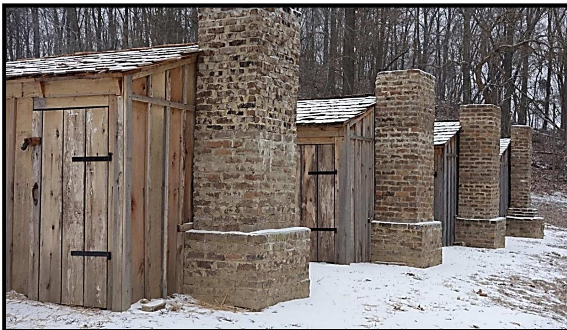
Figure 38: Reconstructed soldier huts, Johnsonville SHP, 2015. Photograph by Author.
