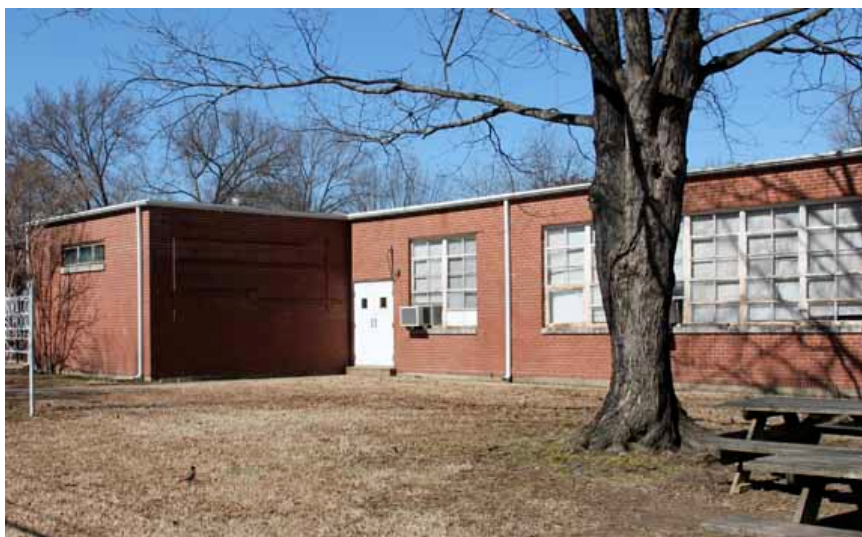
Figure 18. South Elevation of Auxiliary Building, Featuring Secondary Entrance. 2013.
