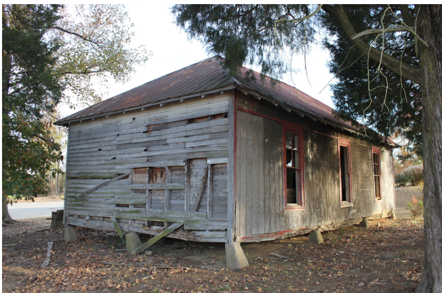
Figure 3. Mt. Zion, North and West Elevations. 2013.
