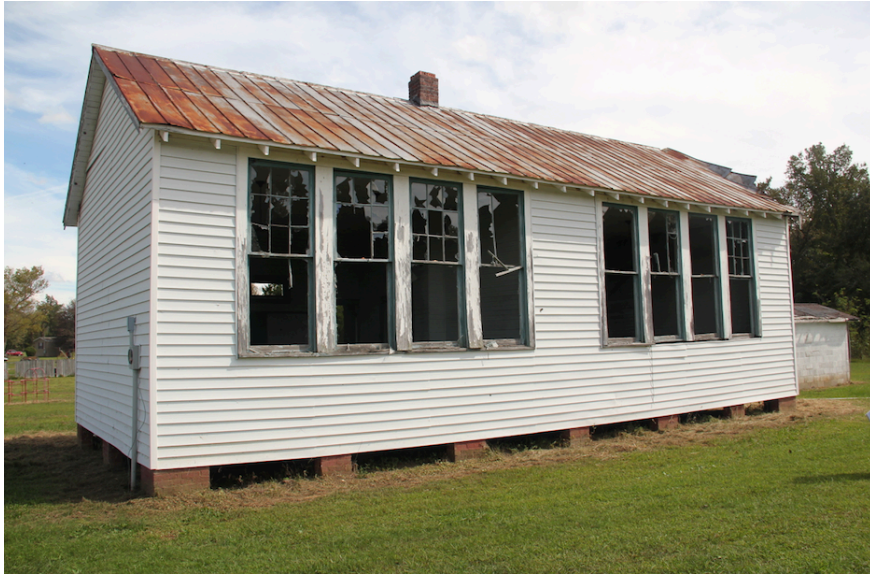
Figure 23. South and West Elevation. 2014.
