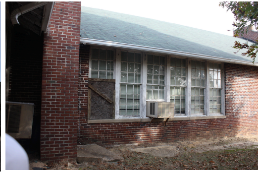
Figure 10.2. West Elevation of South Classroom Wing. Photo Credit: Anne-Leslie Owens. 2010.
