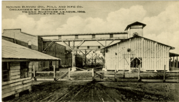
Figure 2.40. Mound Bayou Cotton-Oil Mill. Photograph from archival collection Mound Bayou Historical Preservation Society.
