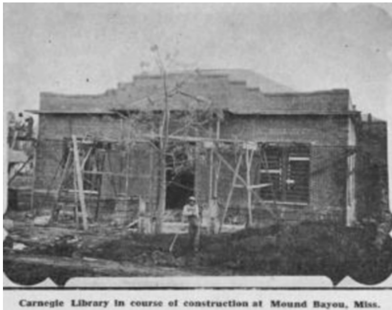
Figure 2.35. Carnegie Library in course of construction at Mound Bayou, Miss. ([1910]). Schomburg Center for Research in Black Culture / General Research and Reference Division. Image ID: 1149612.
