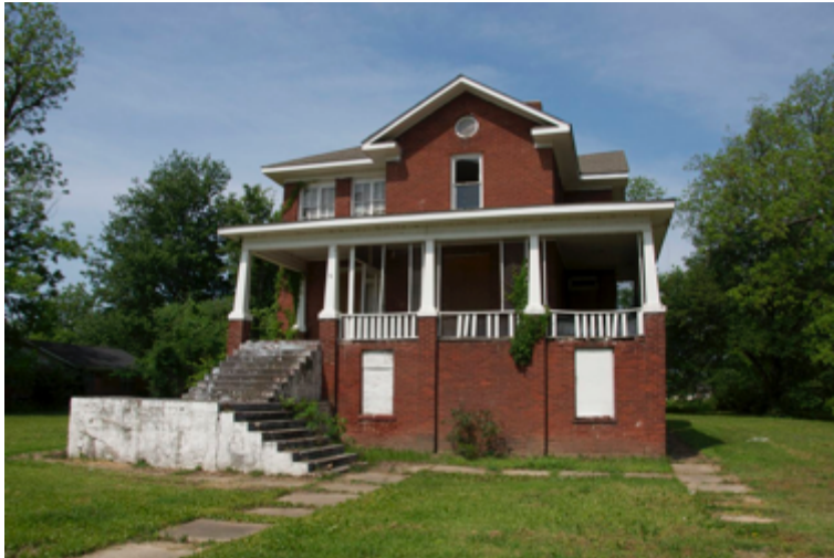
Figure 2.14. Isaiah Montgomery home was built in the Queen Anne style, which was very popular in Mississippi as the railroads expanded between 1880 and 1910. Montgomery's house, with its Square Doric columns, gables, and porch running the width of the house, and partially down one side, must have been an imposing sight when the train passed through. The house faced directly toward the railroad tracks.
