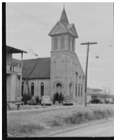
Figure 2.26. AME Church (long exterior view).
