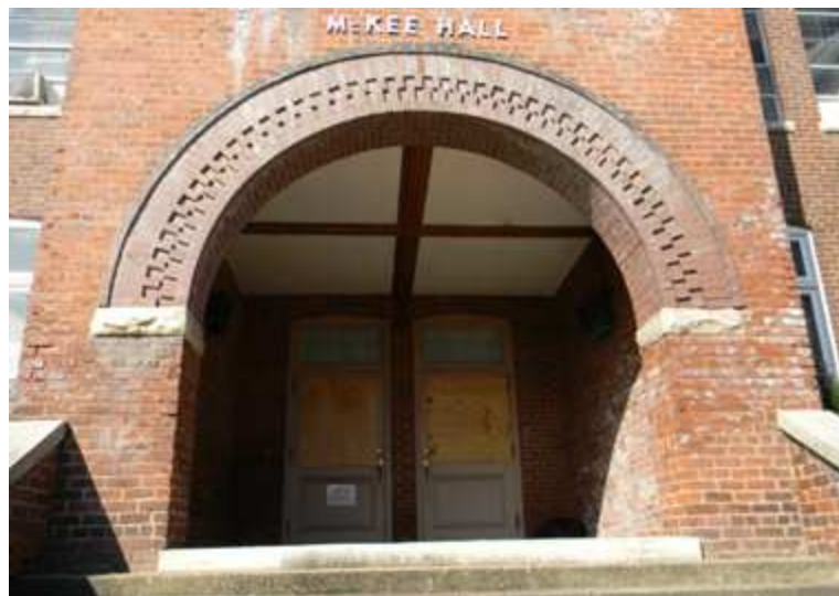
Figure 6. Brick detailing around McKee Hall entryway.
