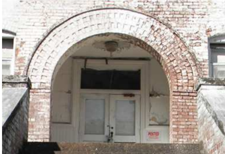
Figure 7. Brick detailing around Elnathan Hall entryway.
