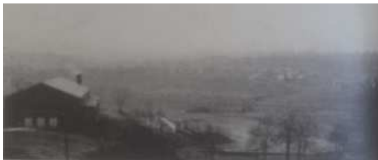
Figure 16. Giffen Memorial Gymnasium and athletic field. 52
