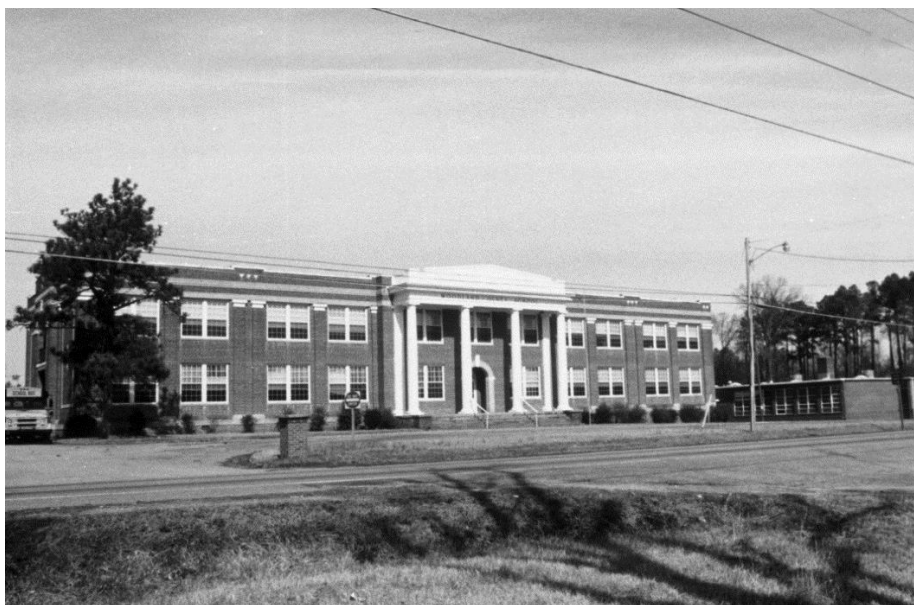
A 18. Woodland-Olney School, Eric Flanagan, architect, Woodland, North Carolina. Photograph by Beth Keane, ca. 1997-2002. Courtesy: State Archives of North Carolina.
