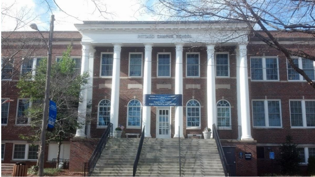
A 1. Homer Pittard Campus School, Marr & Holman, architects, Murfreesboro, Tennessee. Photograph by Matthew T. Norwood, 2014.
