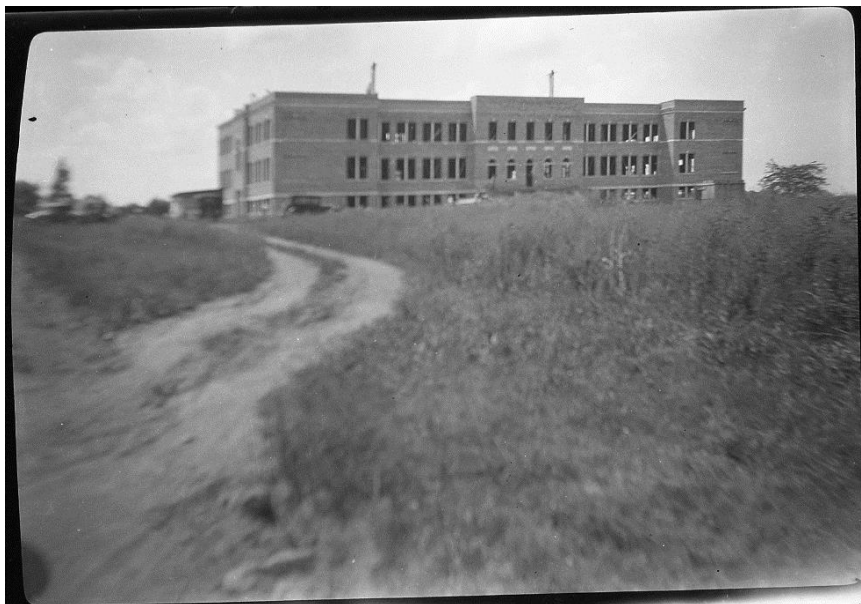
A 3. Homer Pittard Campus School (formerly Training School) under construction, ca. 1928, Marr & Holman, architects, Murfreesboro, Tennessee.
