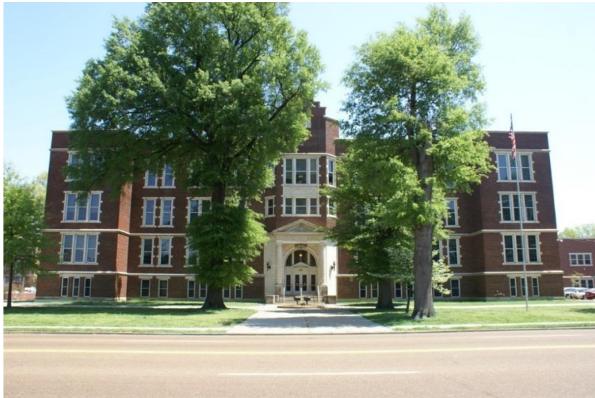
A 14. Central High School, Memphis, Tennessee, B.C. Alsup, architect, Memphis, Tennessee.
