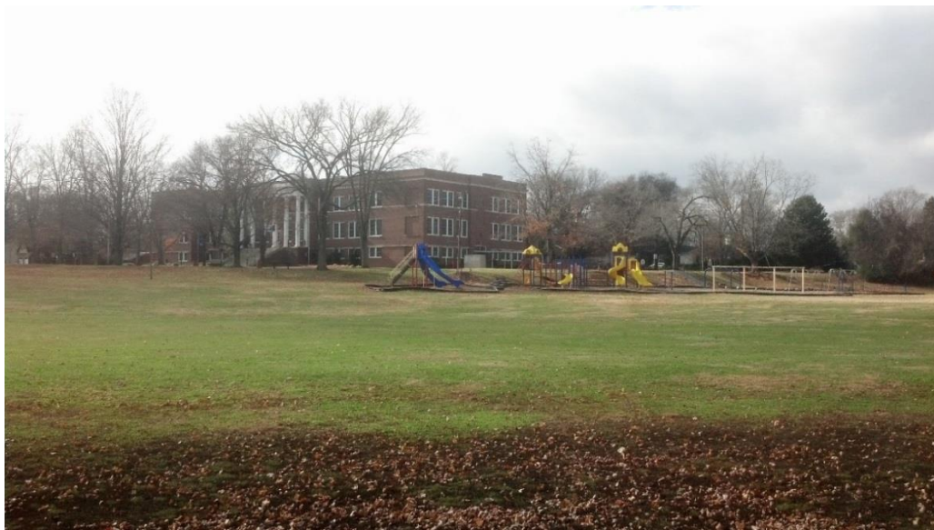
A 2. Homer Pittard Campus School, Marr & Holman, architects, Murfreesboro, Tennessee. Photograph by Matthew T. Norwood, 2014.
