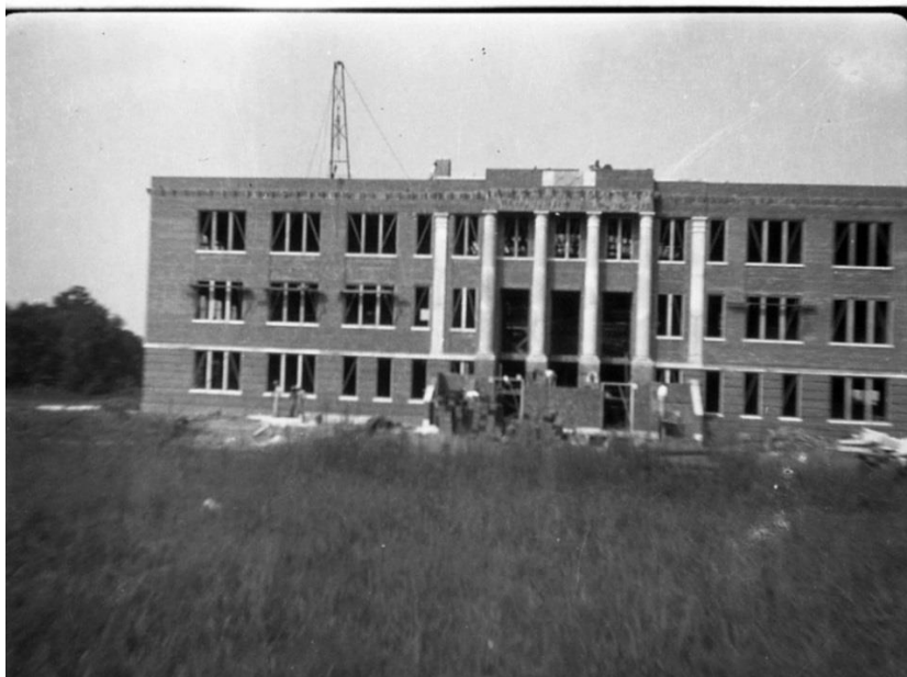
A 4. Homer Pittard Campus School (formerly Training School) under construction, ca 1928, Marr & Holman, architects, Murfreesboro, Tennessee.
