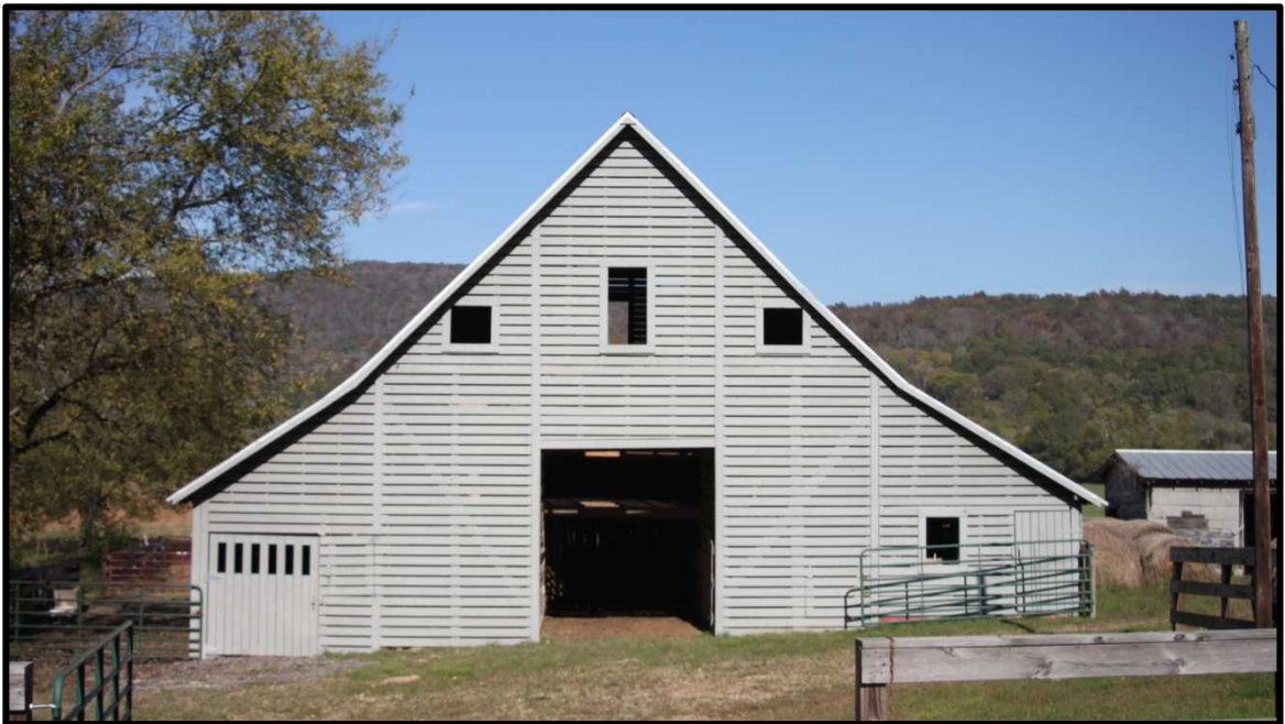
Figure 18: The current renovated barn (Brad Eatherly)
