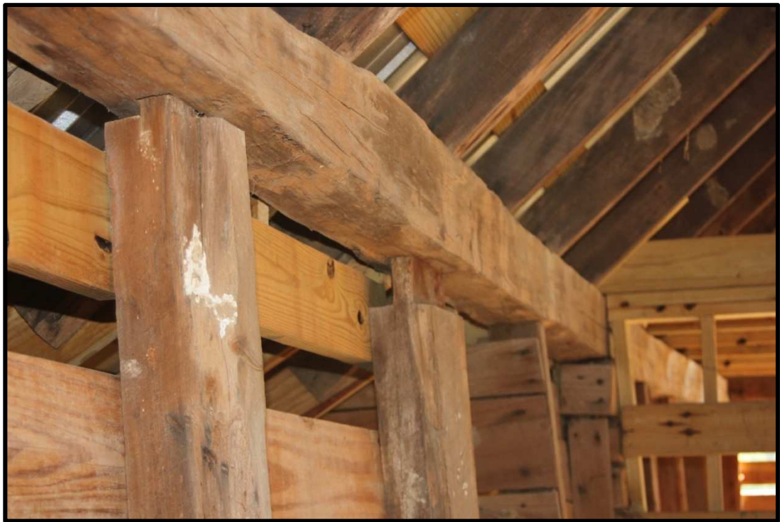
Figure 22: Barn interior-second floor loft's mortise and tenon joints (Brad Eatherly)
