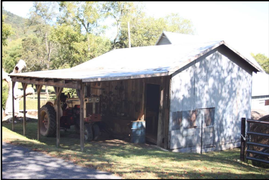
Figure 13: Large equipment and tool shed (Brad Eatherly)
