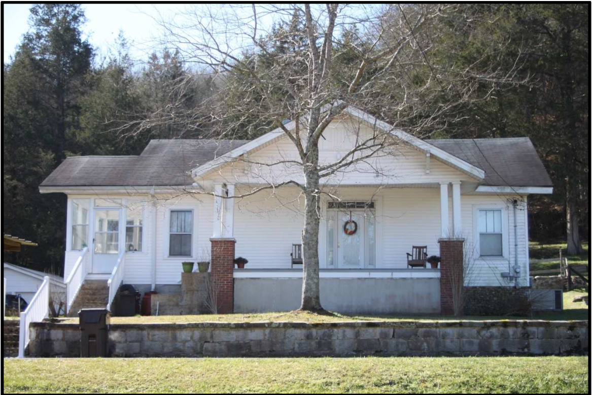
Figure 4: Front façade of the Graham farmhouse (Brad Eatherly)
