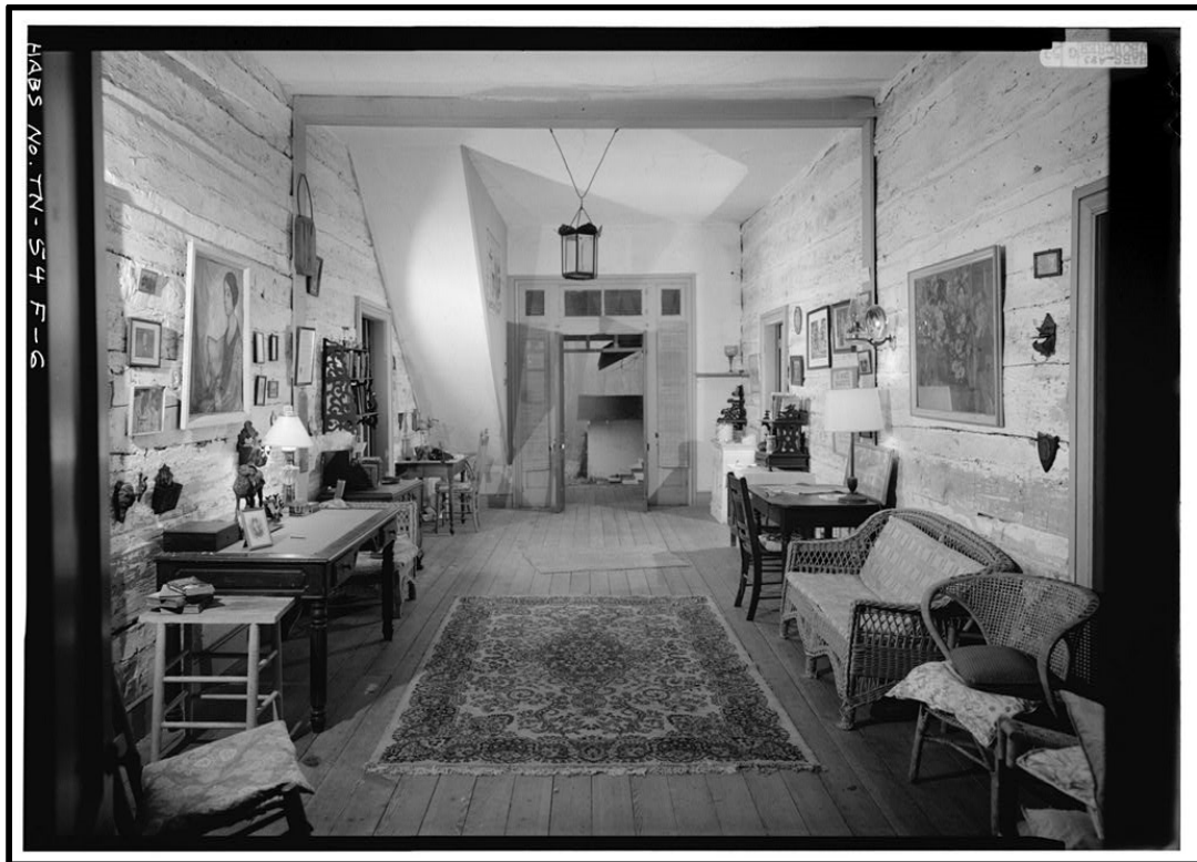
Figure 5: Dog-trot that has been filled in at Old Beersheeba Inn, Beersheeba Springs, TN (HABS)
