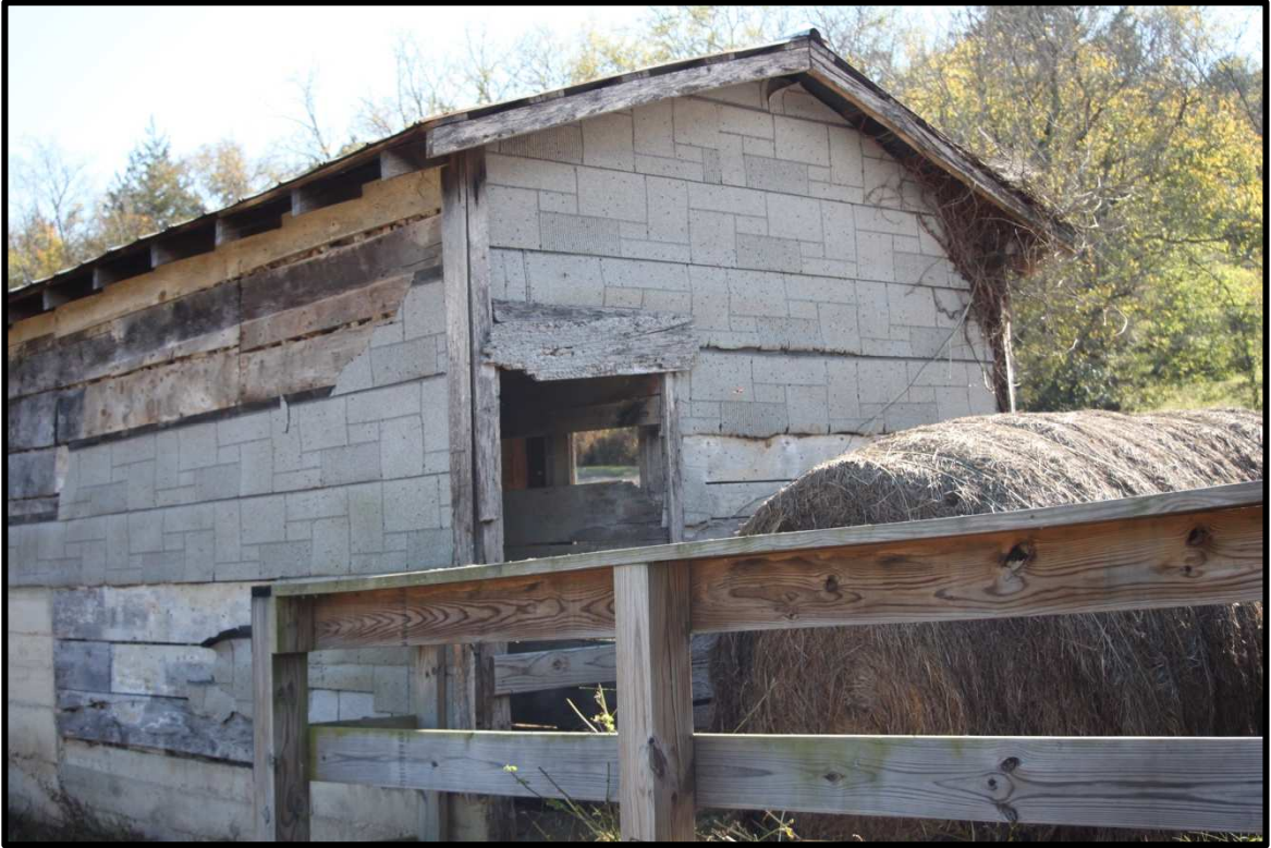
Figure 33: Exterior of farrowing house (Brad Eatherly)
