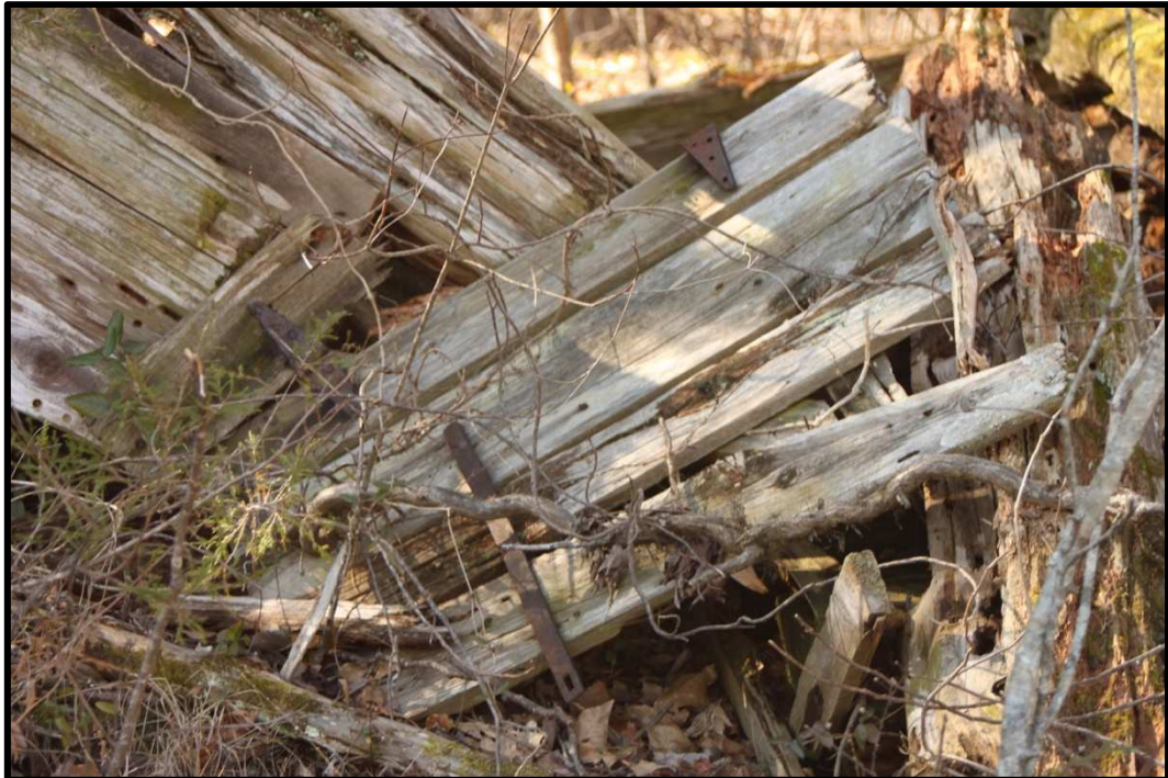
Figure 30: Detail of hardware-two hinges and a locking mechanism (Brad Eatherly)
