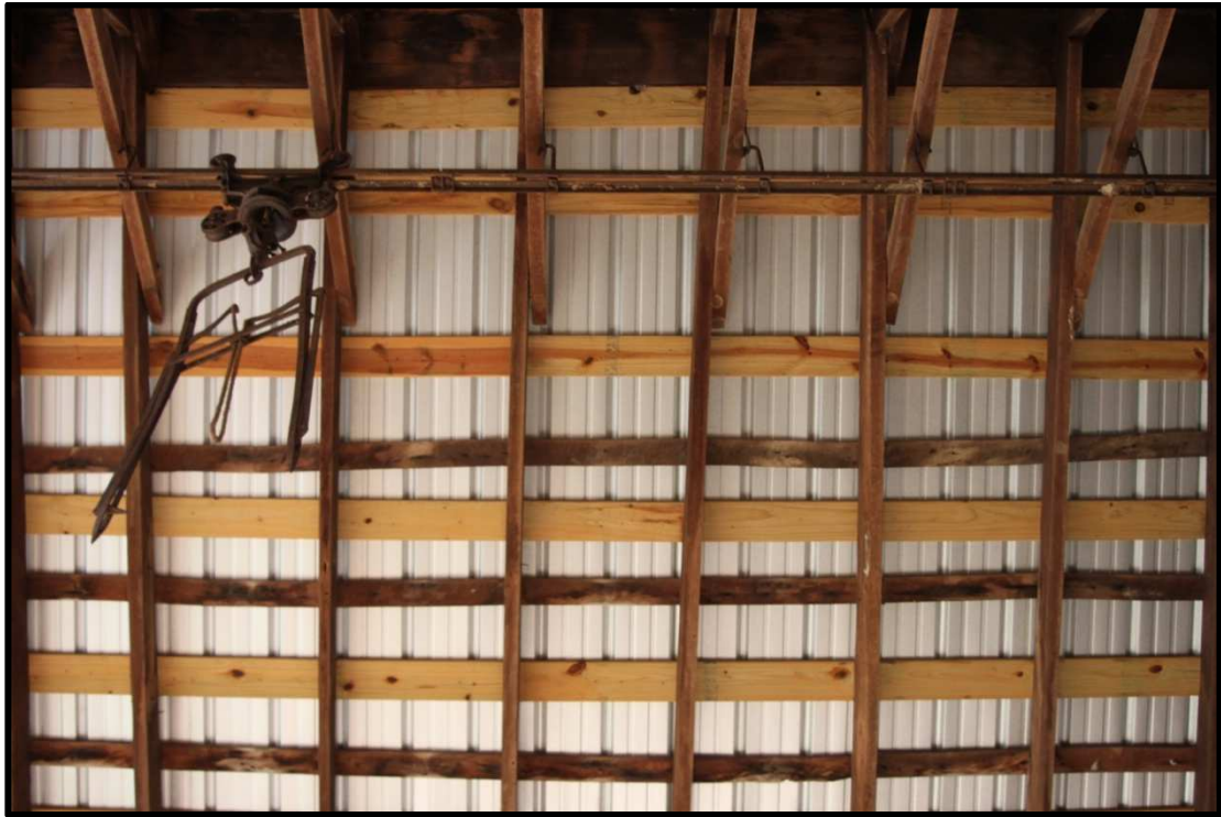
Figure 23: Barn interior-ceiling, with historic wood, new wood, and new tin roof and hay catcher (Brad Eatherly)
