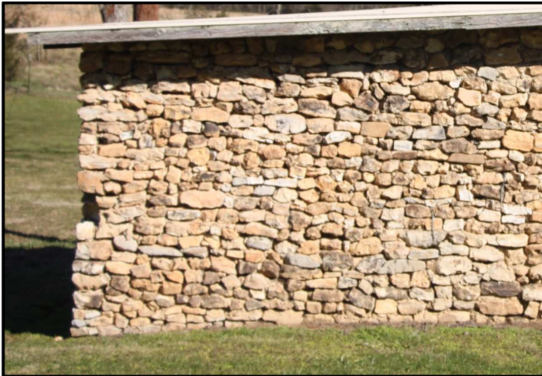
Figure 35: Detail of chicken coop with stones missing in corner (Brad Eatherly)
