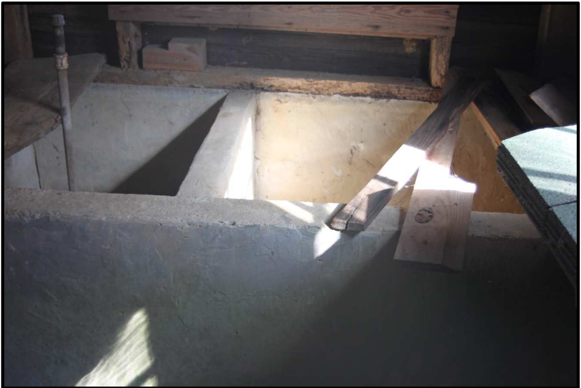
Figure 10: Concrete wash basins within washhouse (Brad Eatherly)
