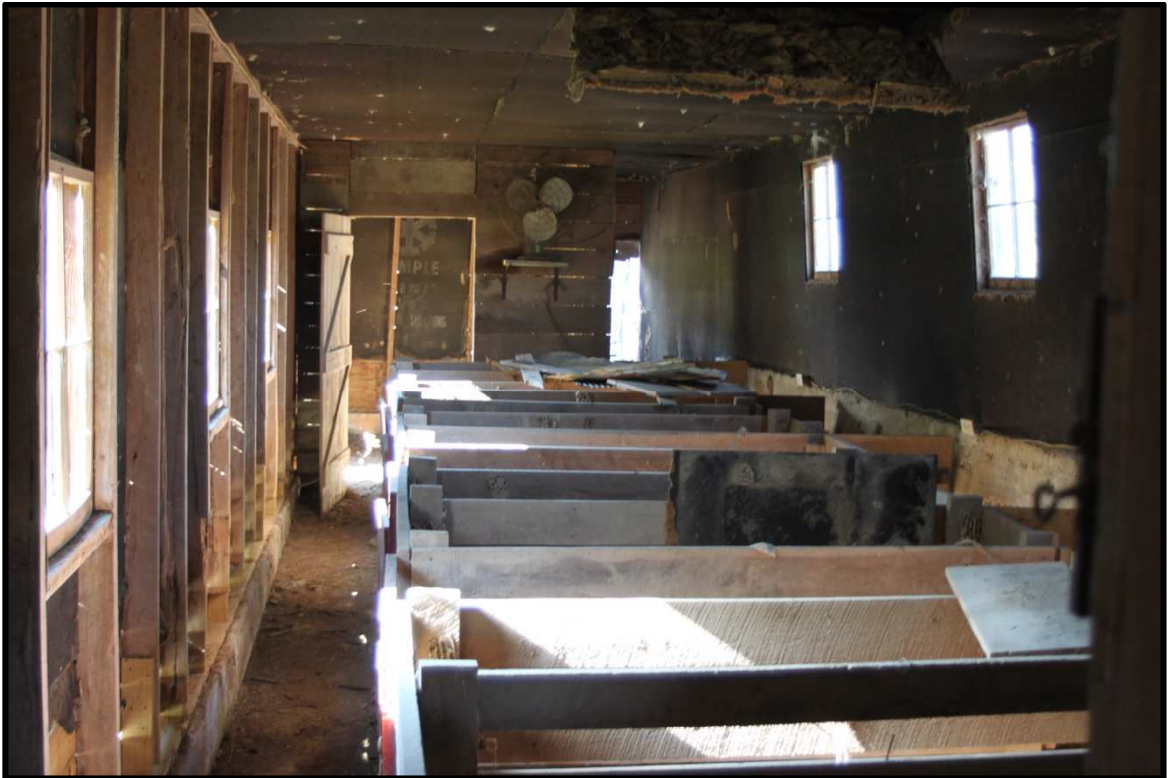
Figure 34: Interior of farrowing house-notice part of the ceiling falling down in foreground (Brad Eatherly)
