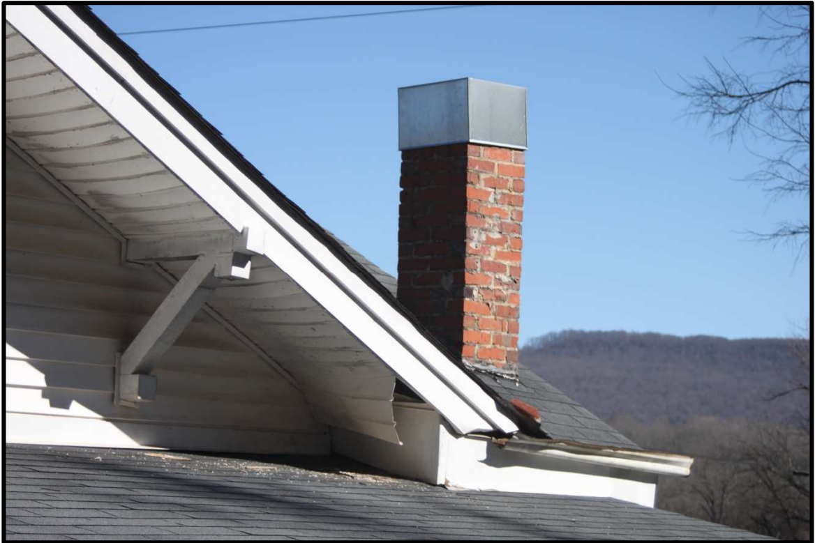
Figure 31: Damage to soffit-notice debris on roof (Brad Eatherly)
