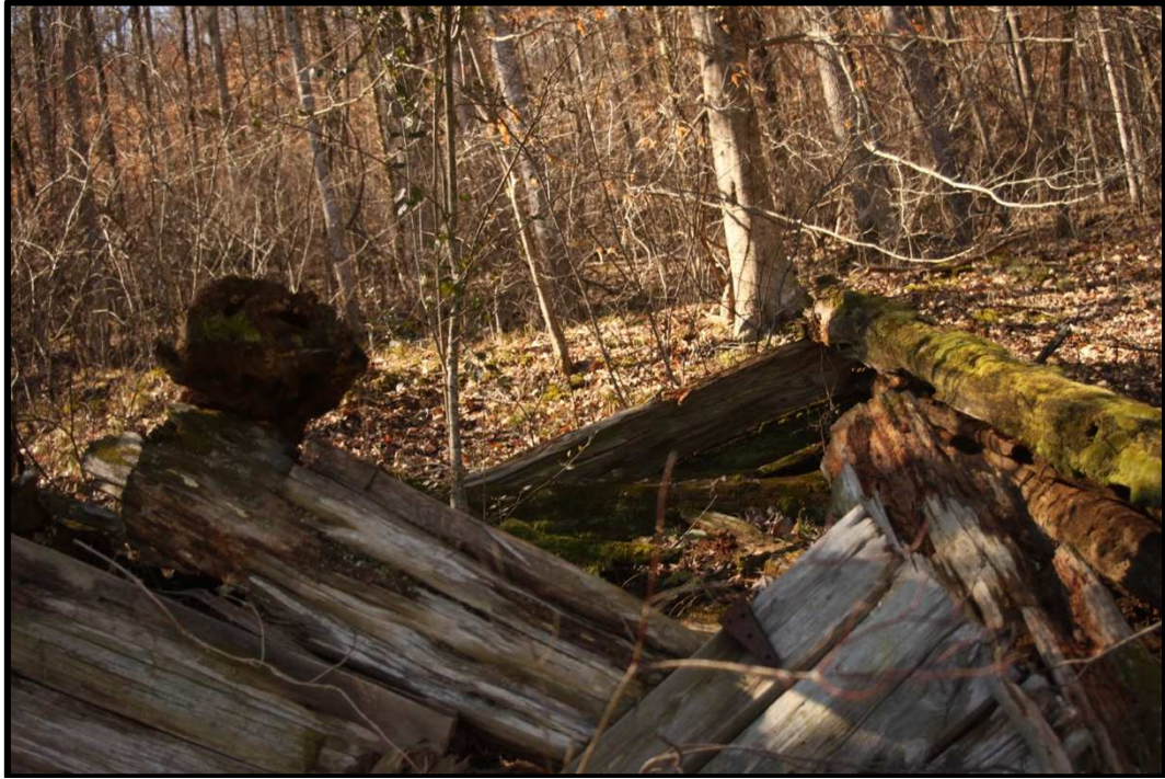
Figure 29: Dilapidated log structure (Brad Eatherly)
