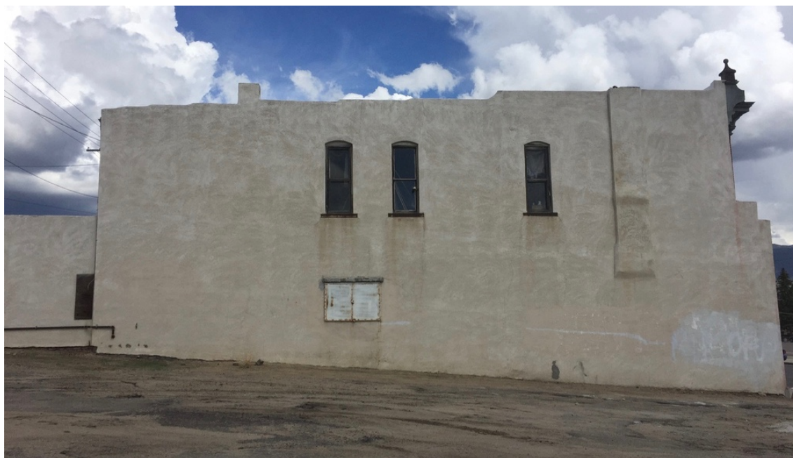
Figure 6. West elevation of original structure, looking east.
