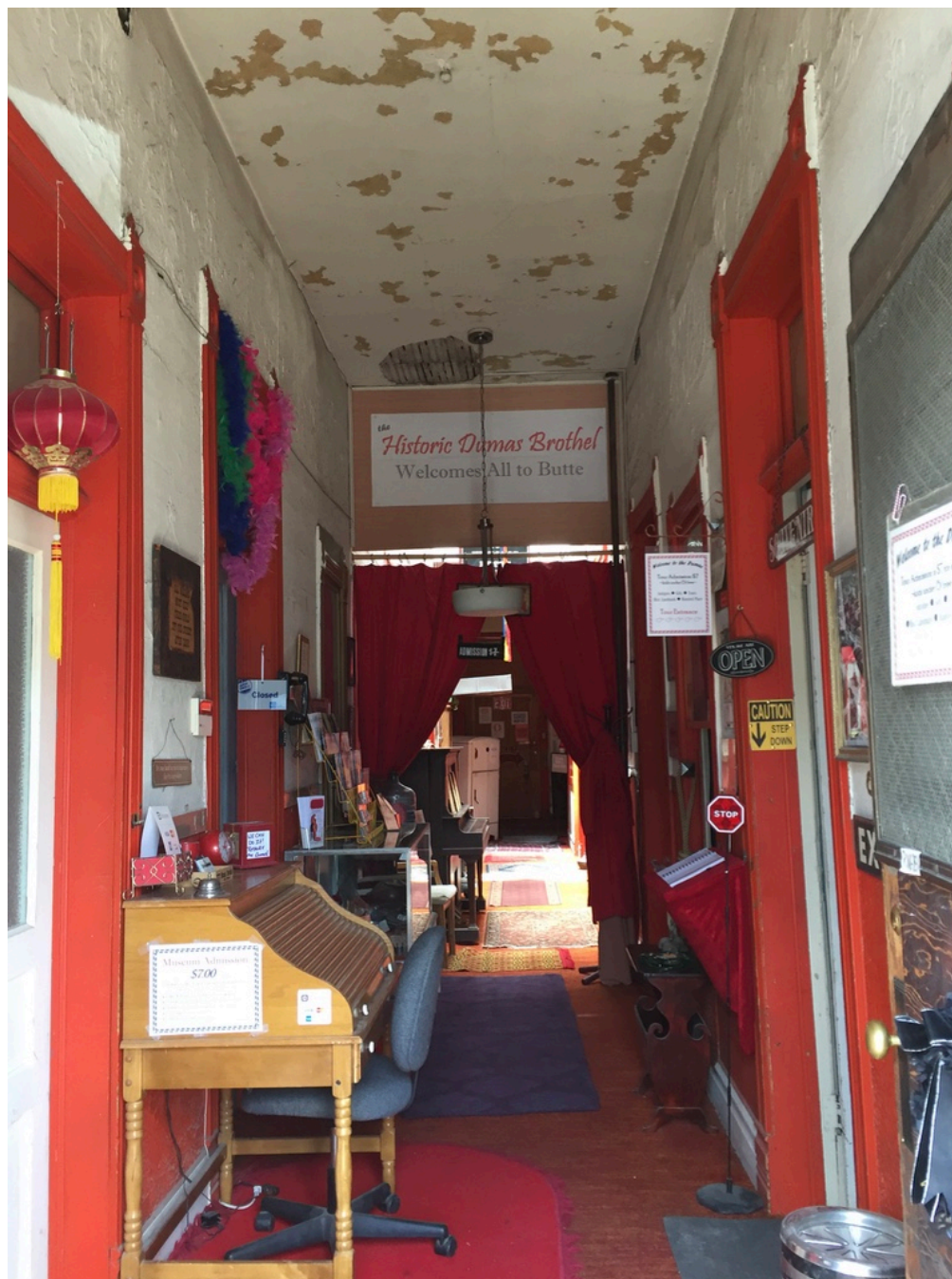
Figure 43. First floor interior, looking north.
