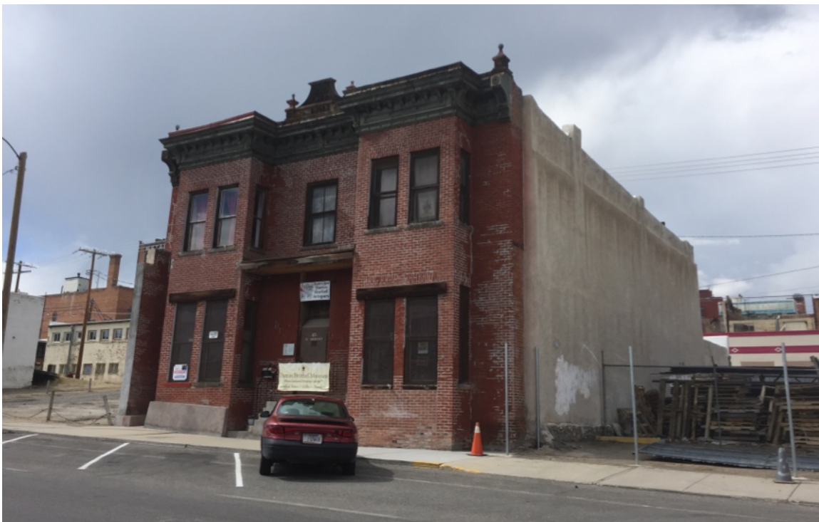
Figure 2. East elevation, looking northwest.
