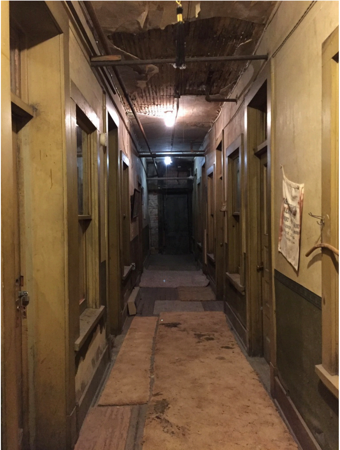
Figure 22. Basement hallway, looking south. Note the window-door pairing and the large door at the end of the hallway.
