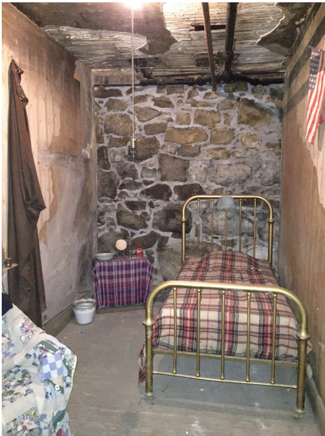
Figure 24. Basement crib, looking west.
