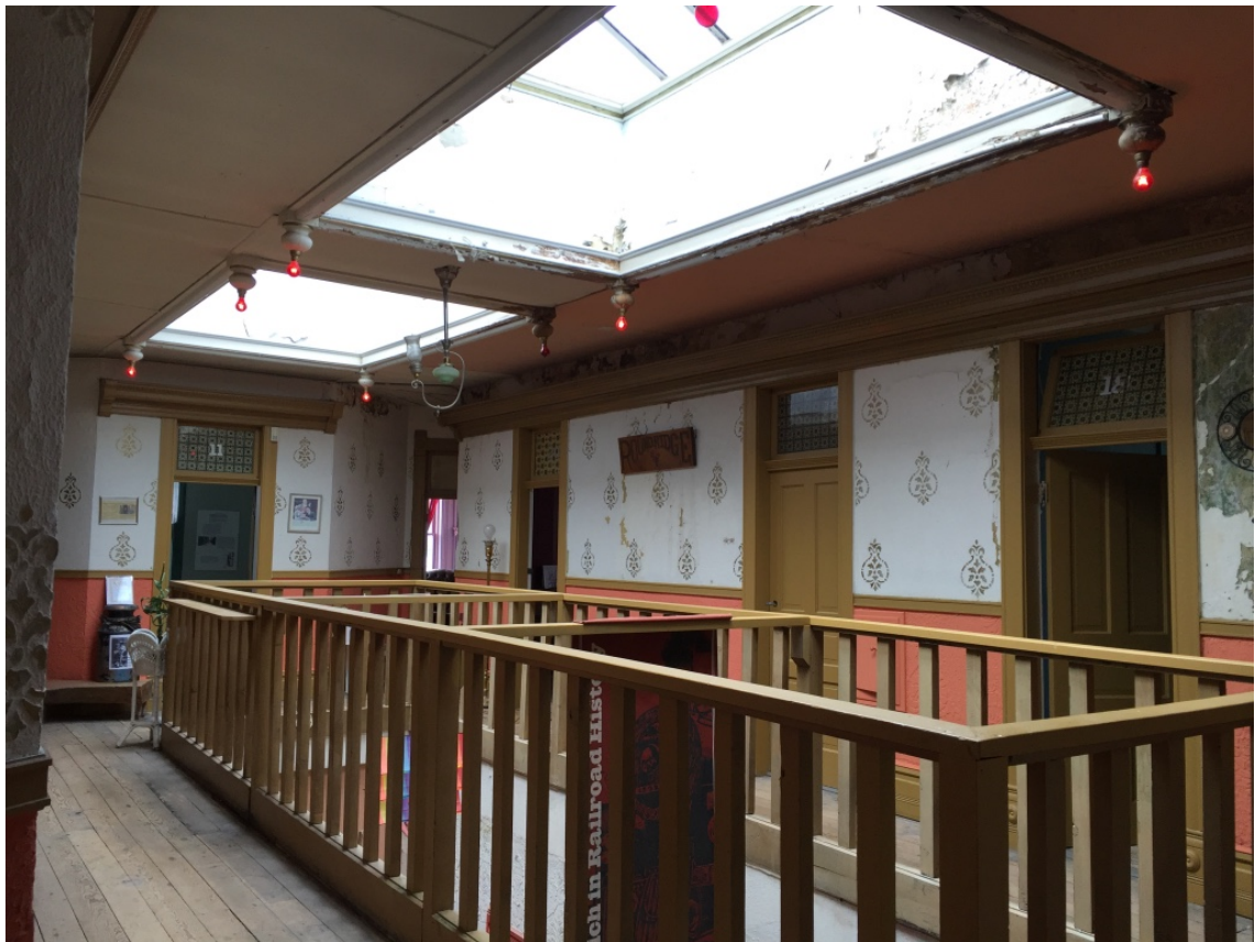
Figure 17. Second floor balcony, looking southwest. Note the embossed walls and wire glass skylights.
