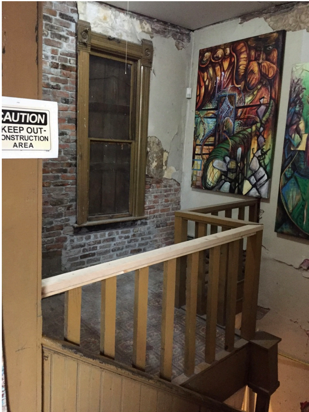
Figure 16. Boarded window at the top of the stairs, looking northeast.
