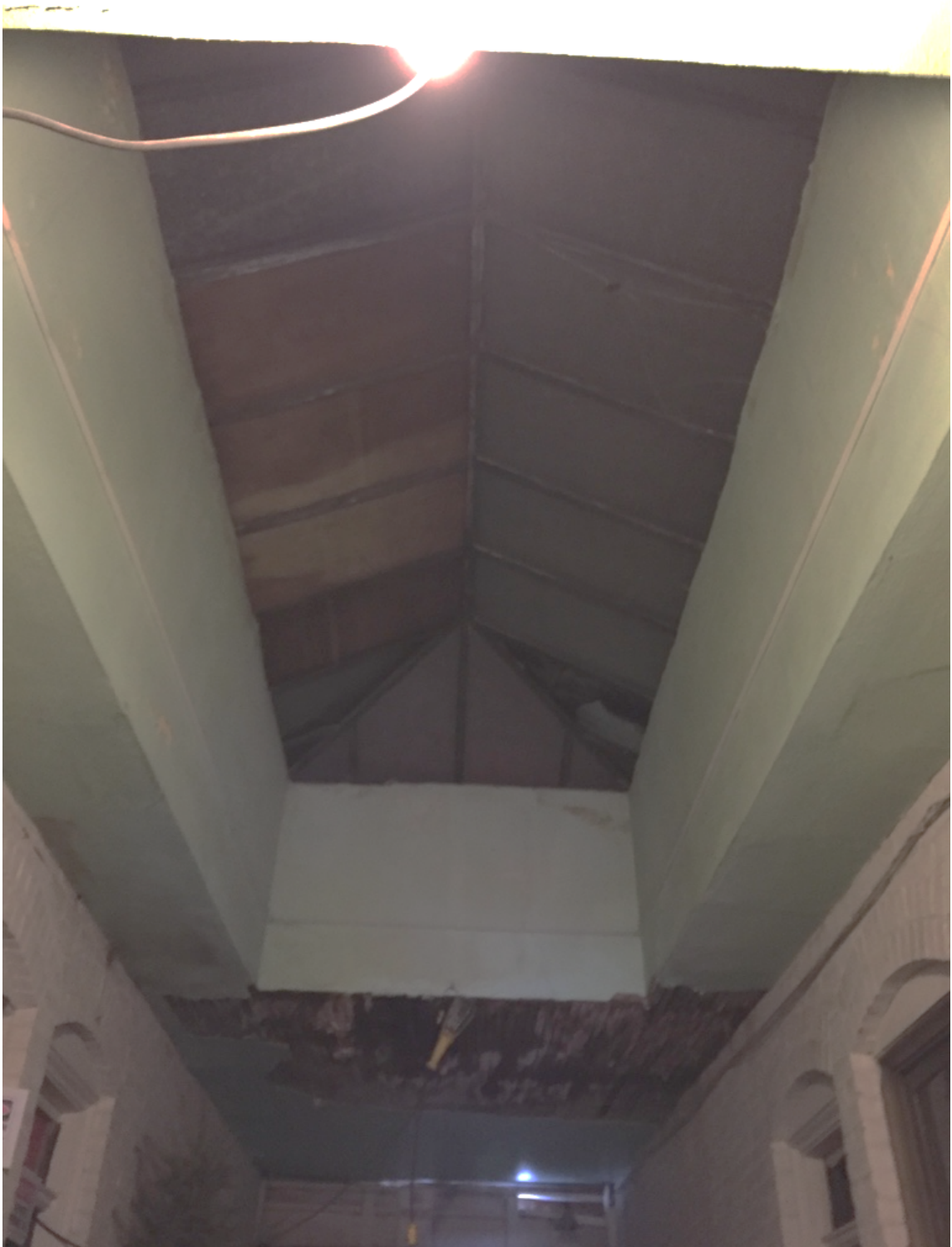
Figure 28. Interior of annex showing covered wire glass skylight.
