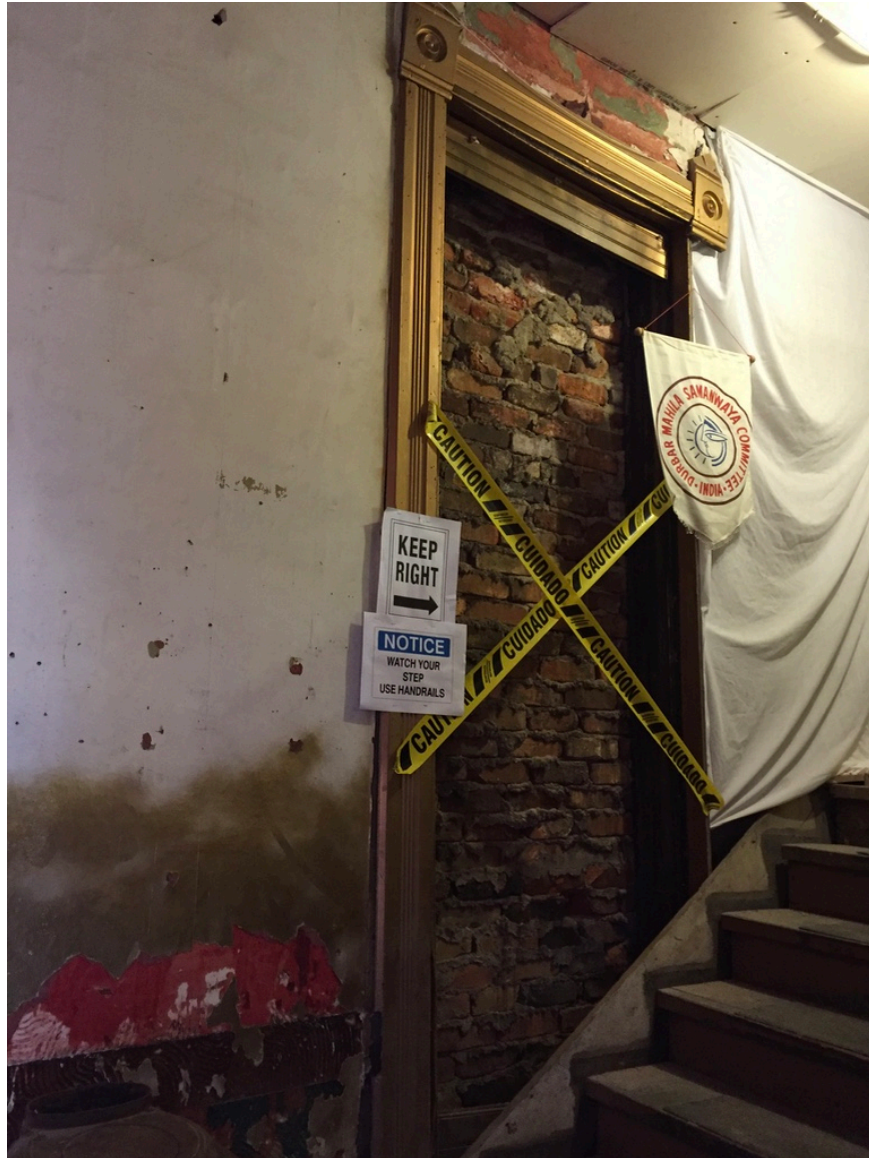
Figure 14. Stairs crossing in front of original rear entrance, looking northeast.
