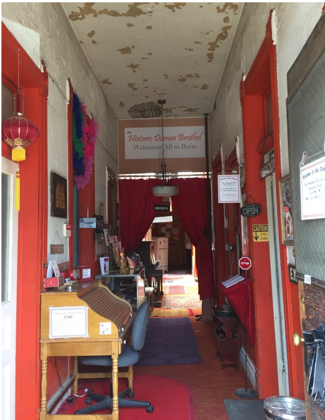
Figure 9. First floor interior, looking north.
