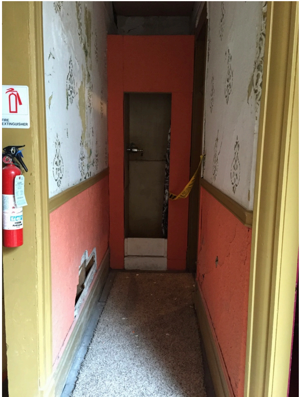
Figure 15. Shower stall at the top of the stairs, looking west.
