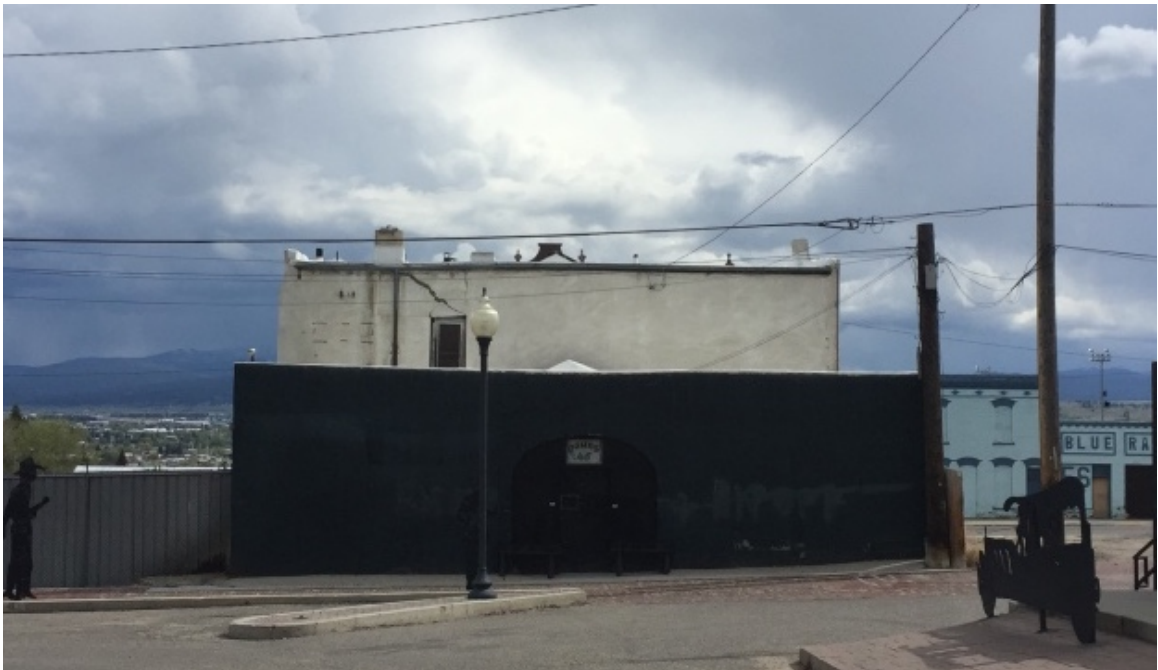
Figure 5. North elevation, looking south.
