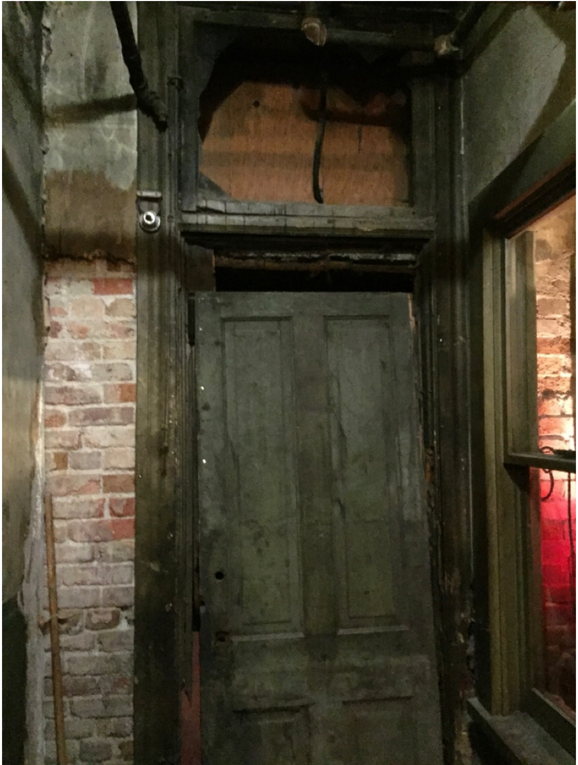
Figure 23. Detail of metal door at the end of the basement hallway, looking south. This would have opened to a tunnel, which was filled in decades ago. Note the transom window.
