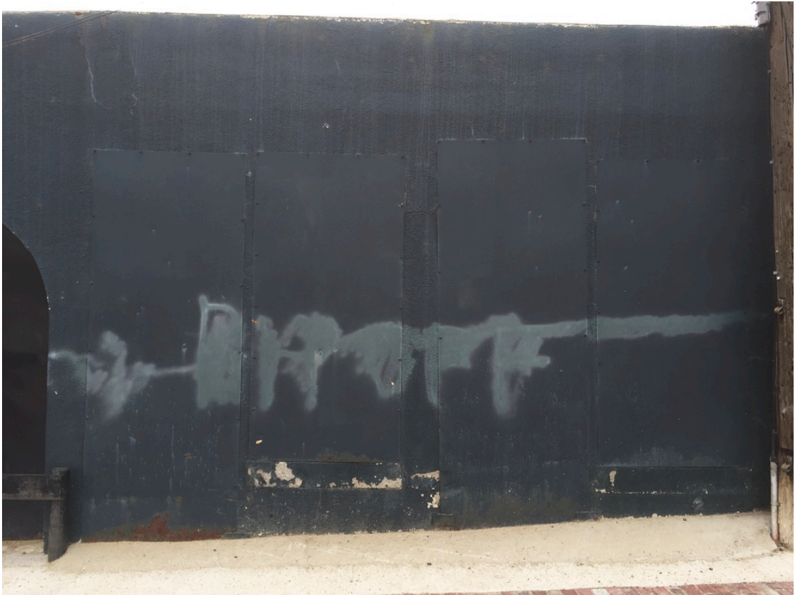
Figure 4. Covered crib doors and windows. North elevation, looking south.
