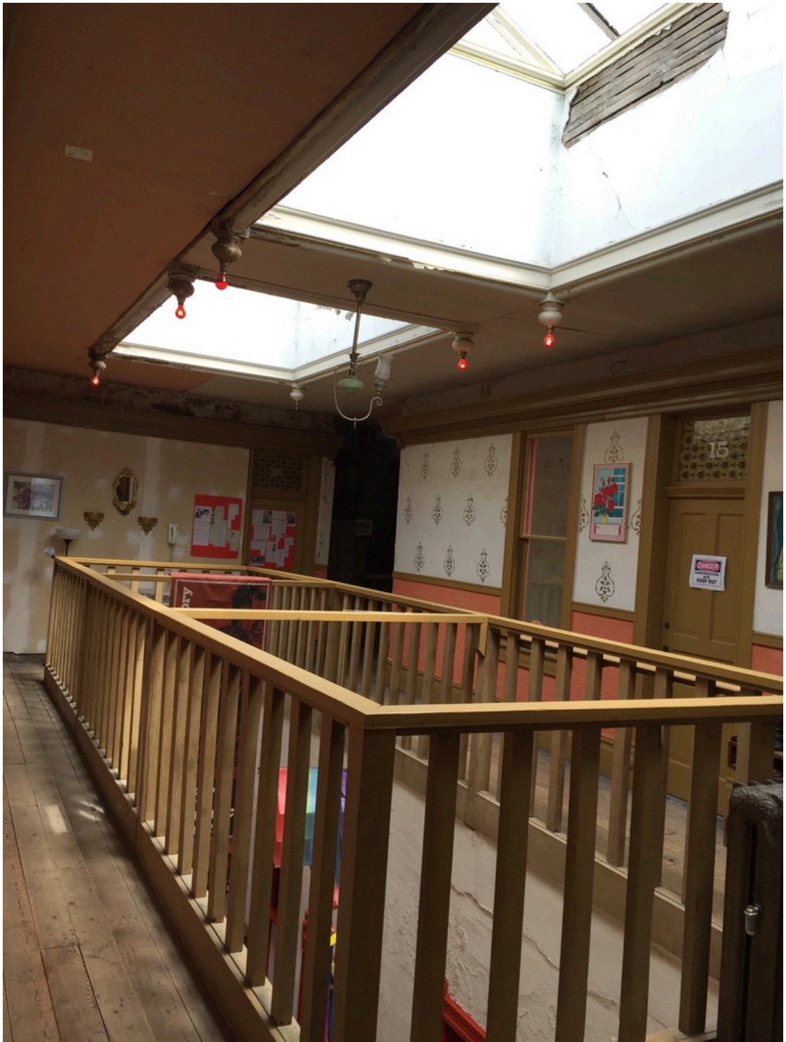
Figure 18. Second floor balcony, looking northeast. Note the windows to the right of the balcony and the new drywall on the far wall.
