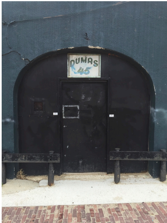
Figure 3. Rear entry. North elevation, looking south.
