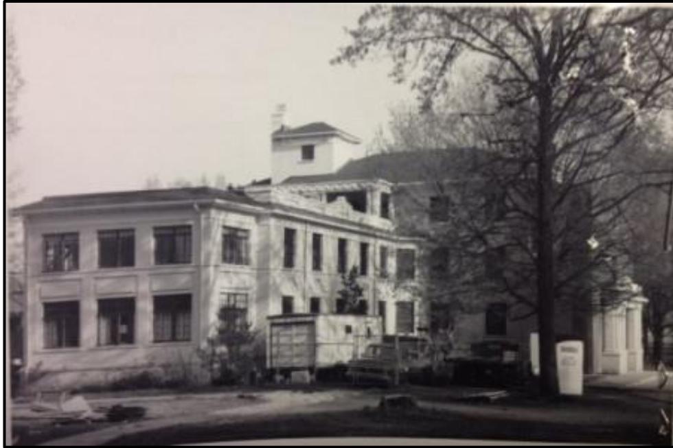
Figure 38. Administration Building, Julius Marks Sanatorium, Kentucky Historic Resources Inventory Survey, 1983.
