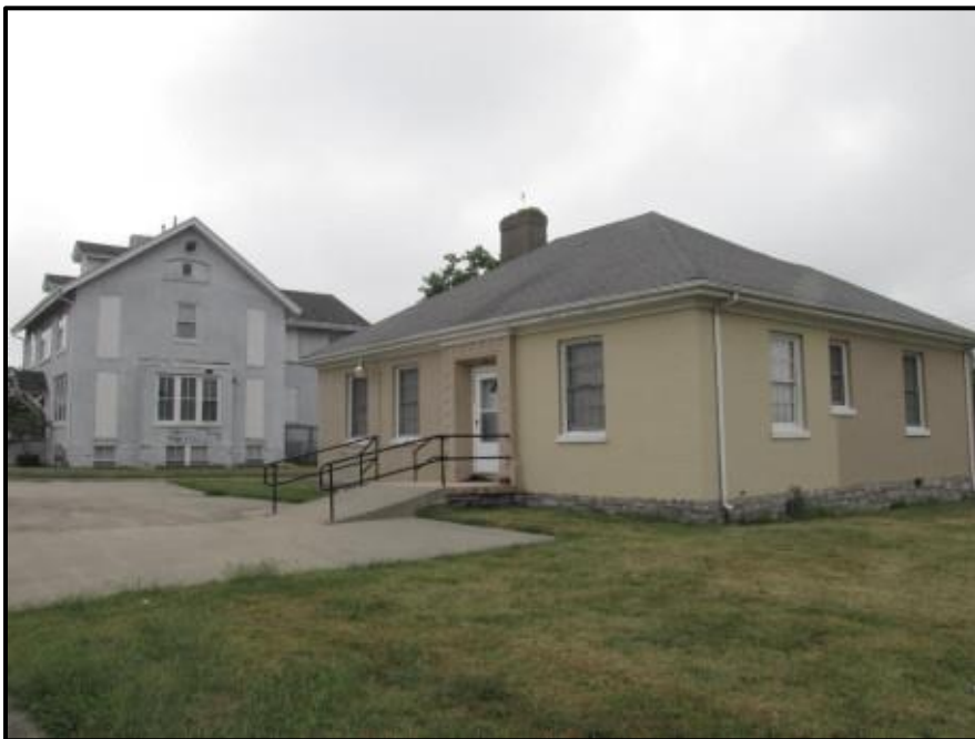
Figure 46. Nurse's Quarters and Storage Building, Julius Marks Sanatorium, 2015, Photograph by Author.
