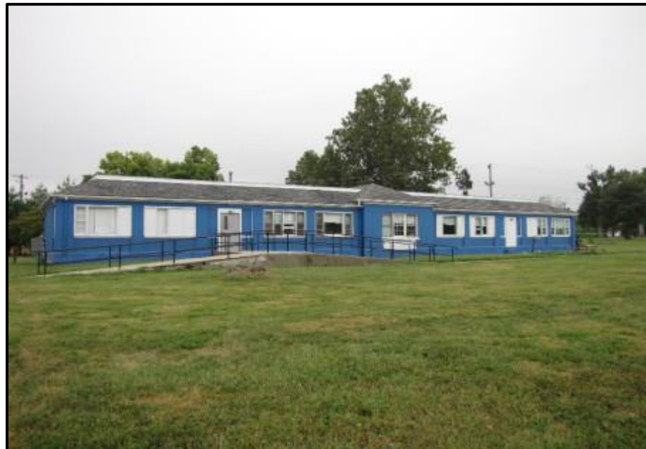
Figure 50. South Ambulatory (Sleeping Pavilion/ Patient Cottage), 2015, Photograph by Author.
