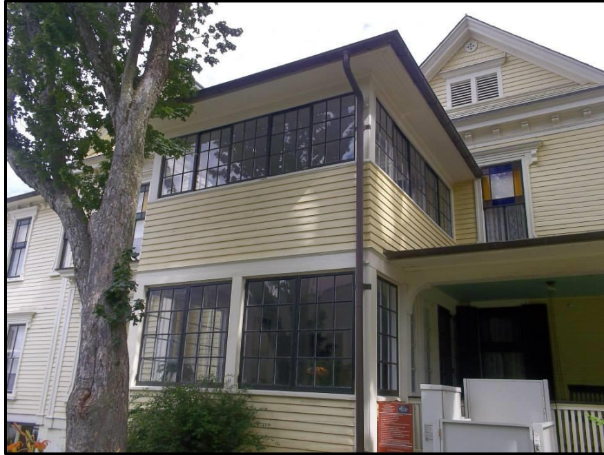
Figure 30. Sleeping Porch and Sun Parlor Side Addition, Thomas Wolfe Memorial, Asheville, NC, Photograph by Author.
