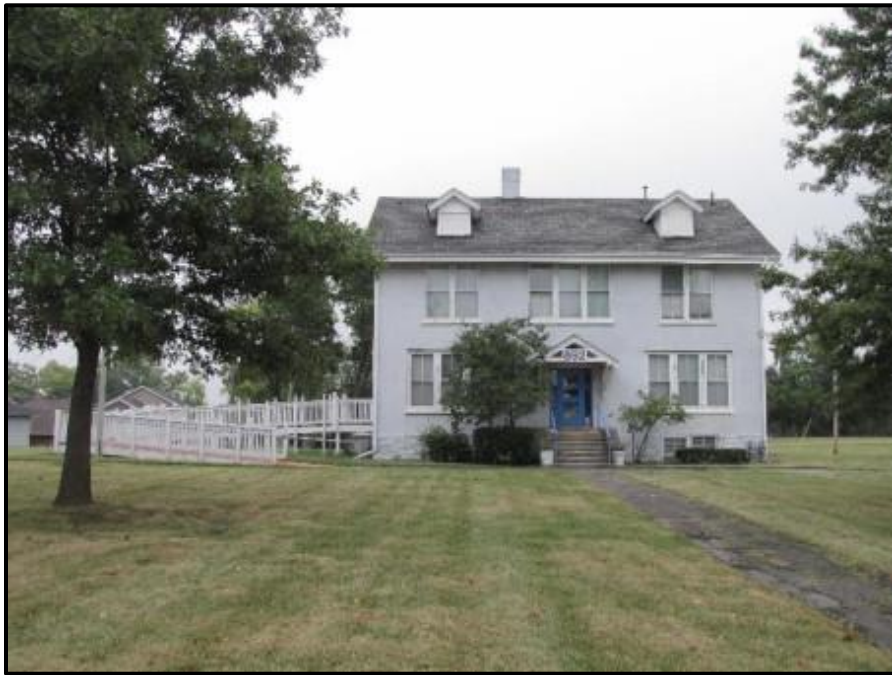
Figure 44. Nurse's Quarters, Julius Marks Sanatorium, 2015, Photograph by Author.
