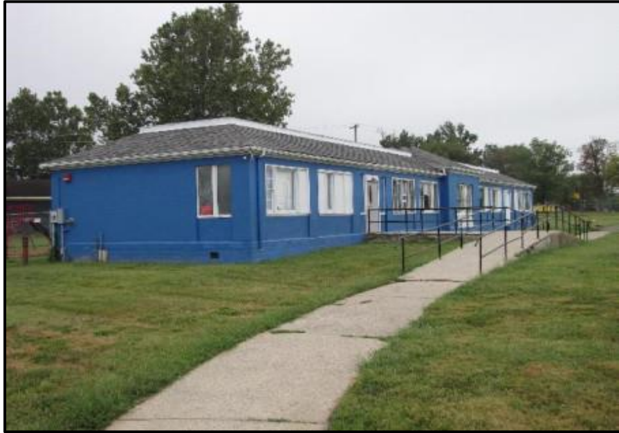
Figure 49. South Ambulatory (Sleeping Pavilion/ Patient Cottage), 2015, Photograph by Author.
