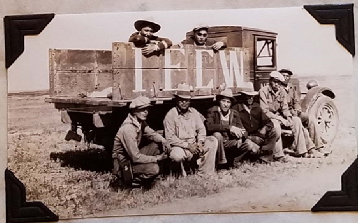
Figure 11, IECW Truck and Crew. Photo 6: RG 75 Box 106 CCC-ID General Records 1933-1944 Fort Peck, NARA, Washington, D.C.
