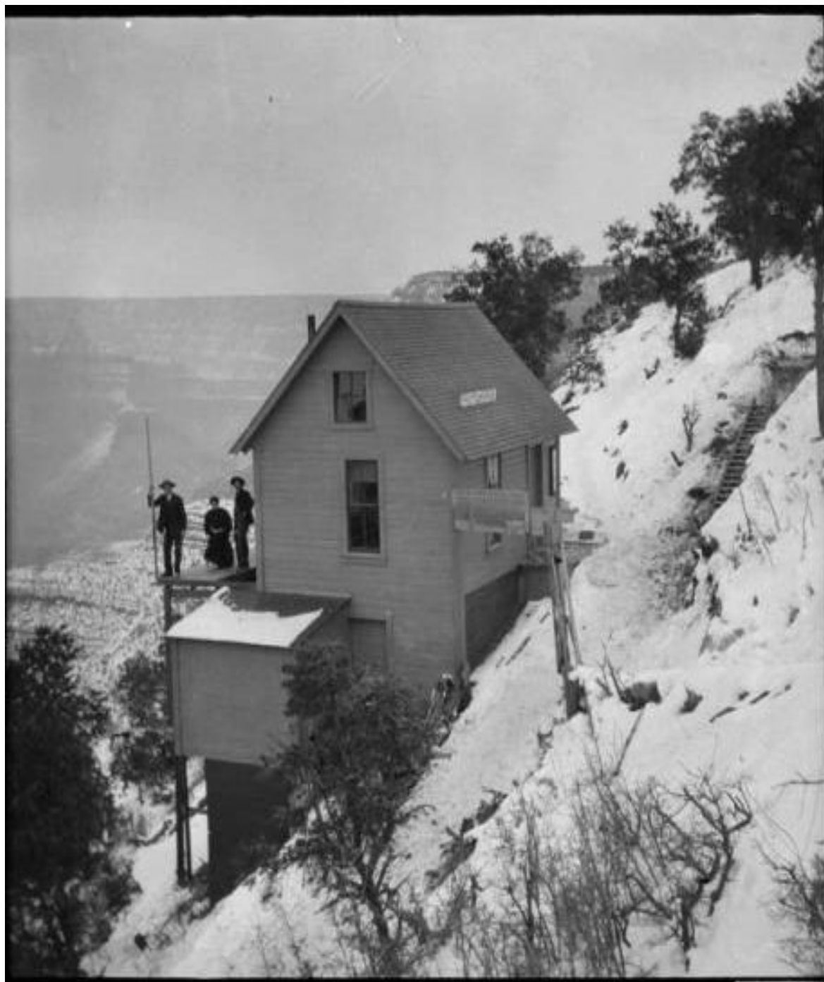
Figure 5: Kolb Studio addition under construction, circa 1906. Courtesy of Kolb Collection.
