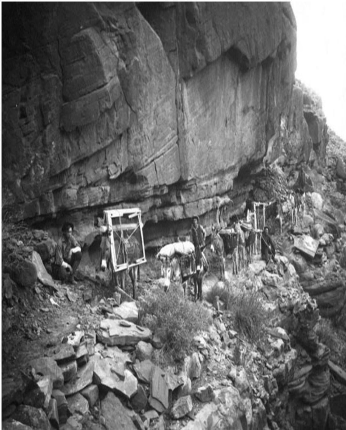
Figure 6: The Kolb Brothers went to great lengths to collect water and make money off the mule-riding industry including packing building materials to construct their inner-canyon darkroom. Courtesy of Kolb Collection.
