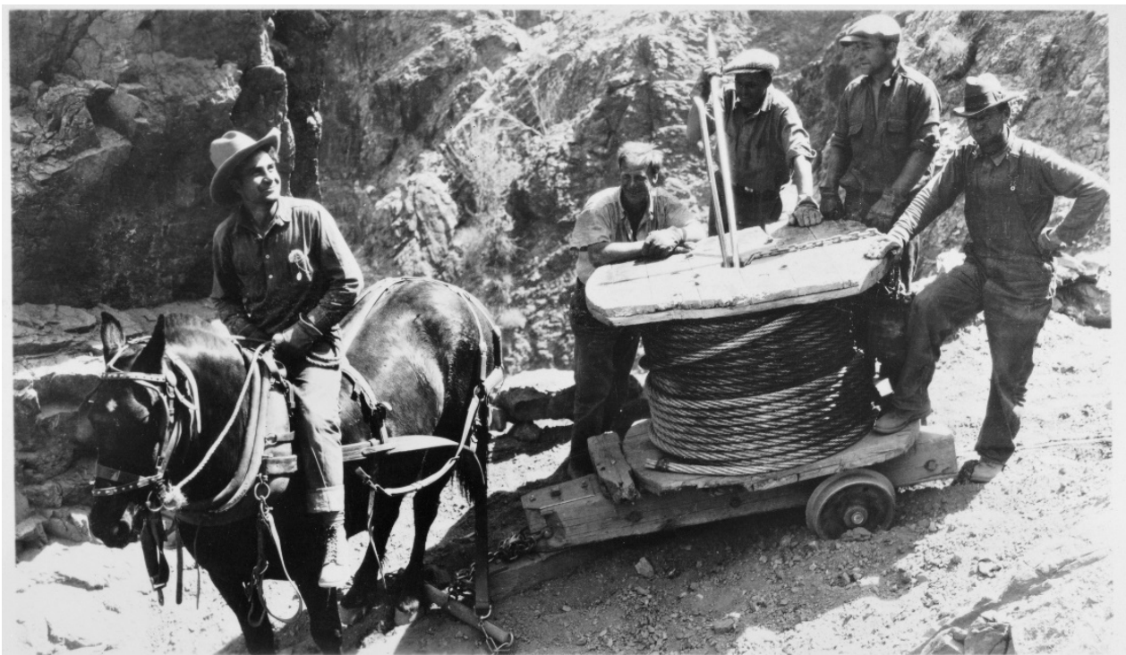
Figure 12: Crews built specially designed sleds to aid in transporting coils of steel cable. Courtesy of Library of Congress.
