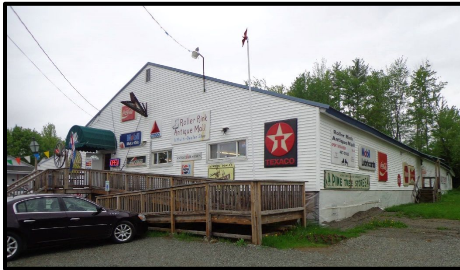
Figure 5.1: Exterior of Roller Rink Antique Mall, Roller Rink Antique Mall Facebook Page, June 13, 2013. 1
