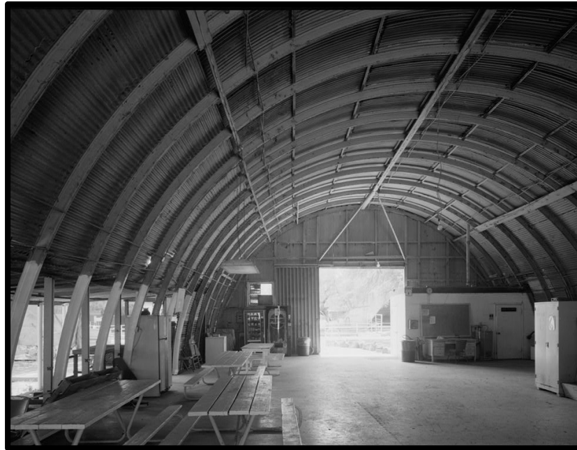
Figure 3.45: “Facility 1520, Interior of Quonset Hut, View Facing West. -Naval Air Station Barbers Point, Quonset Hut Type 1 – 40’x 100’, Between John F. Kennedy & Harrison Streets, South of Bismarck Sea Road, Ewa, Honolulu County, HI,” Historic American Buildings Survey Collection, Prints and Photographs Division, Library of Congress.
