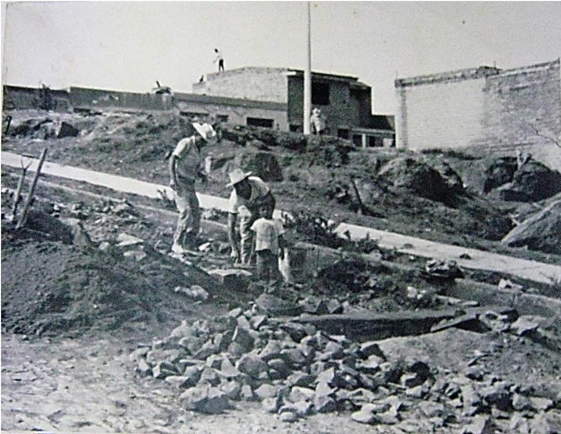
Figure 1.11. Two men working on the earliest stages of constructing a house in Santa Cecilia in 1968, while a young boy stares at the camera. Notice the slant down to the right side of the photo, toward Oblatos Canyon. Above and behind them is the main street Joaquin Amaro Avenue. Photo used by permission from Centros Educativos Oblatos.
